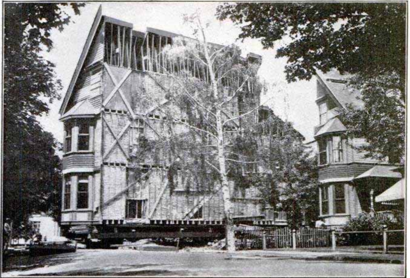
Moving a House by Cutting It in Halves and Taking It to New Location in Two Loads
