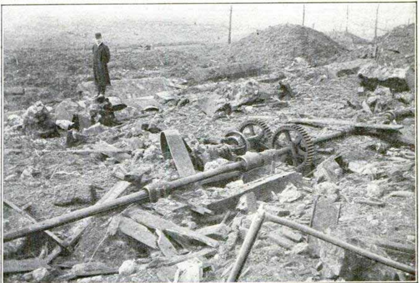
Exact Spot where the Pleasant Prairie Explosion Started; All that Remained of the Glazing Mill, where 1,000 Pounds of Powder was Ignited by Some Agency, Probably Friction
