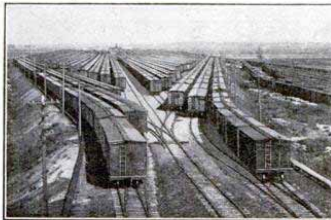
The Cars on the Tracks, Sorted without a Switch Engine and without Risk to Life or Limb, Ready to Go Direct to the Railroads Which Are to Take Them from Chicago
