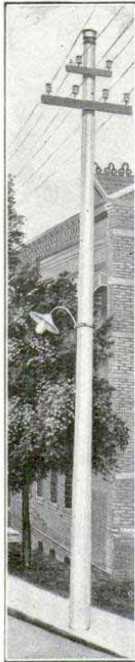
Hollow Concrete Pole Which Was Cast by the New Centrifugal Process
