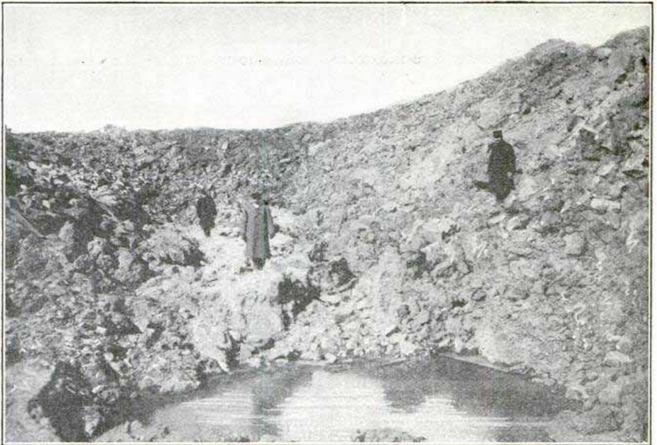
This Hole, All that Marks the Spot where One of the Powder Magazines Stood at Pleasant Prairie, Wis., is about 150 Feet Long, and 50 Feet Deep at One End. Great Lumps of Hard Clay Cling to the Sides of the Hole
