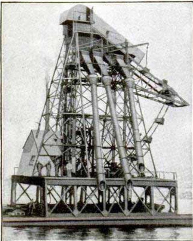
New Type of Ship-Coaling Tower Constructed at Southampton, Eng.
