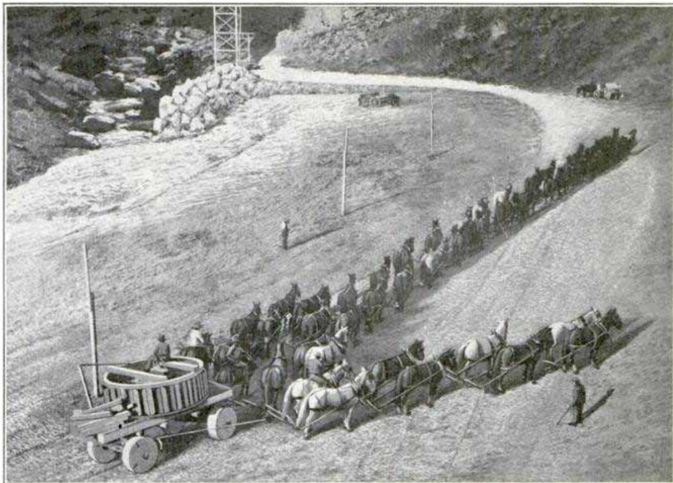
48-Horse Team Hauling Machinery for a California Electric-Generating Station
