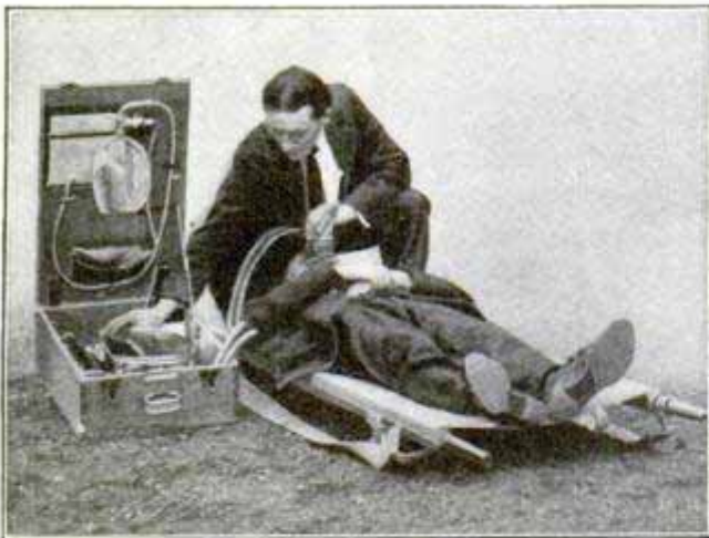
The Pulmotor at Work near One of the Rescue Cars
