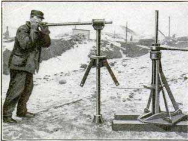
The Jack by Which the Man is Standing is the Type Used through the Holes in the Bottom of the Tank. The Jack at the Right is the Type Used at the Rim.
