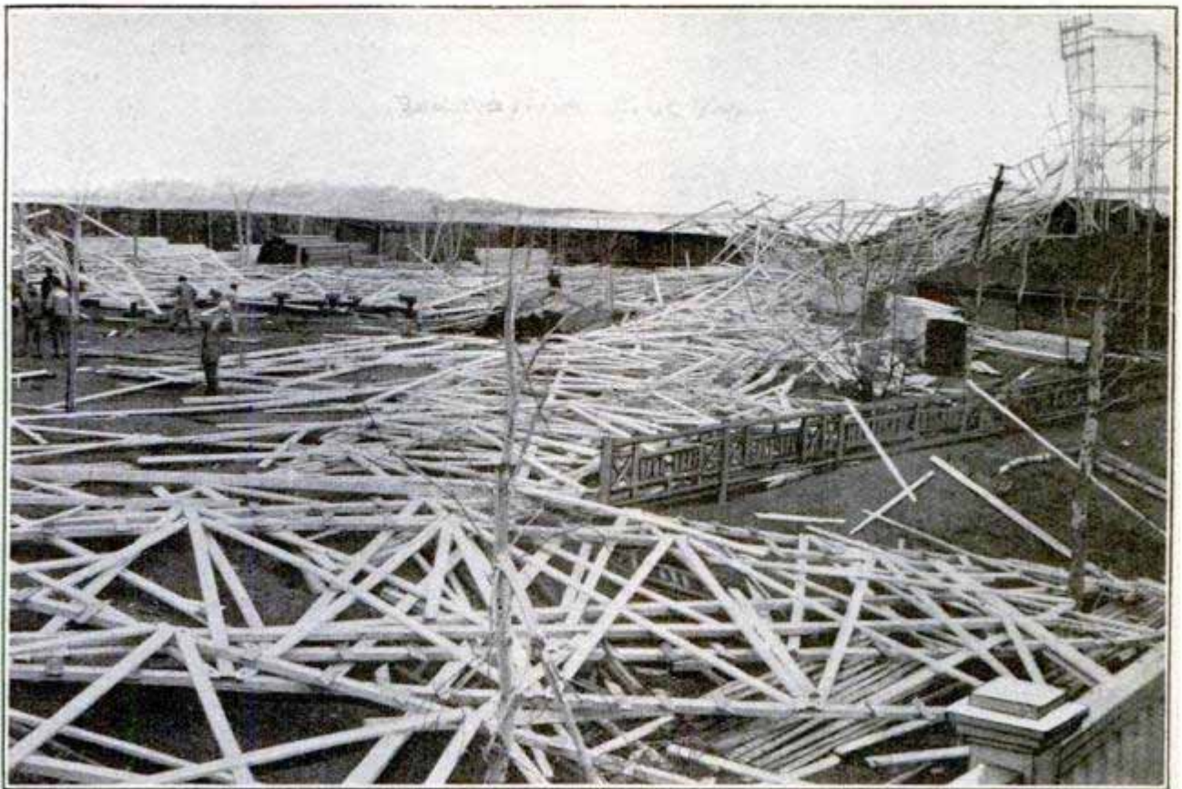
Ruins of the Giant Scenic Railway Wrecked by Wind at Denver. Fell Like so Many Dominoes
