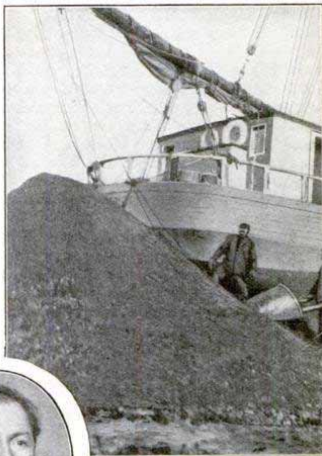
Digging the Schooner Out of the Sands —Note Improved Steam Shovel at Right
