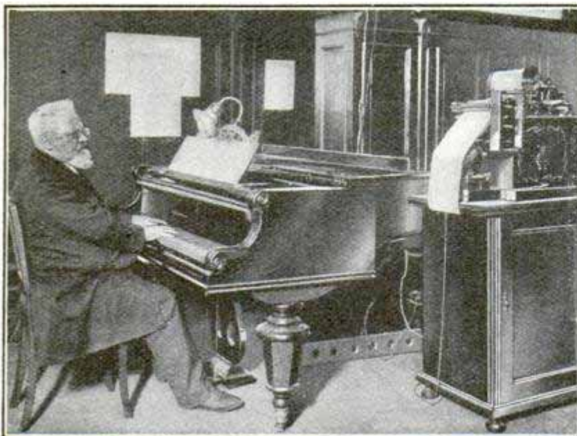
The "Kromarograph," a Music-Recording Machine Invented by a German Composer
