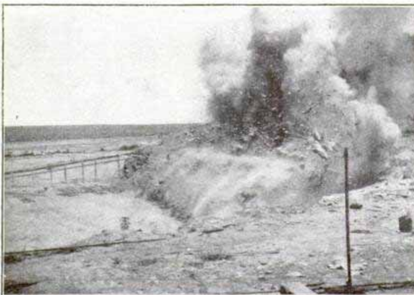
Photograph Made at the Instant a Charge of 1,200 Lb. of Dynamite was Exploded
