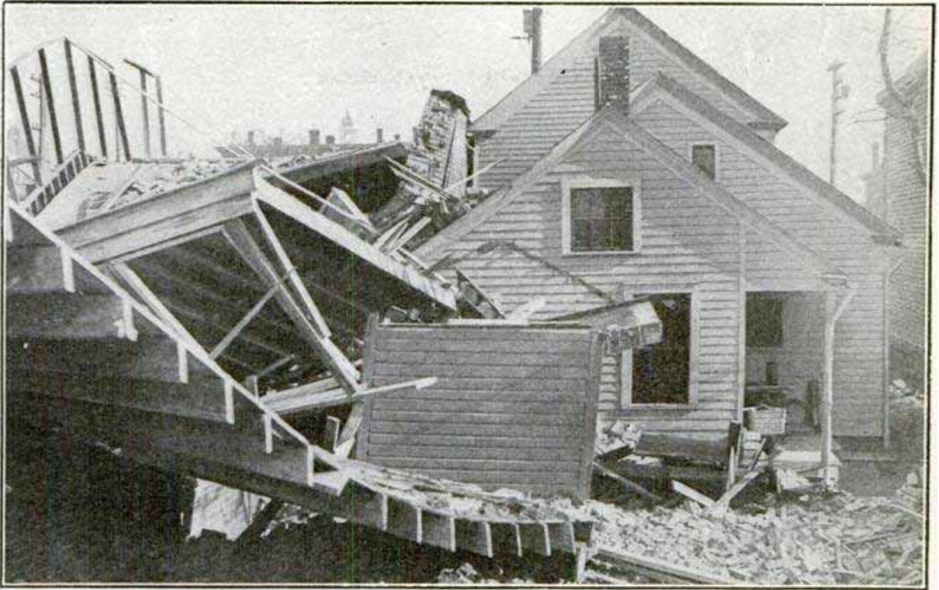
The Persons Killed and Injured Were Eating Supper in the Small Wooden Building Adjoining When the Concrete Structure Collapsed
