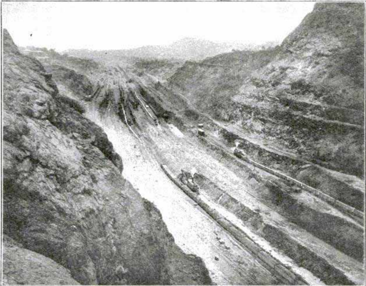
THE CULEBRA CUT, LOOKING NORTH
