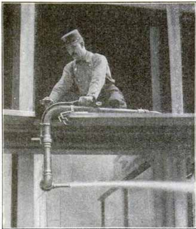
Operating a Deluge Pipe
