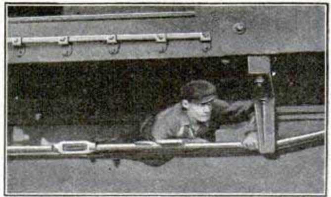
Across a Plank Between the Rods—Gritty and Perilous
