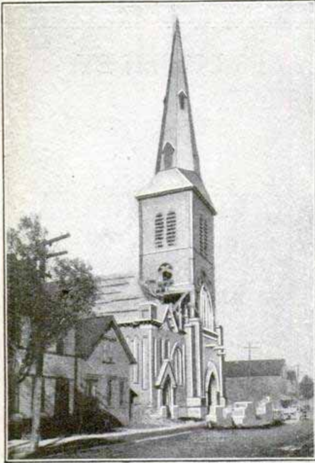
Constructing New Church Under an Old Steeple
