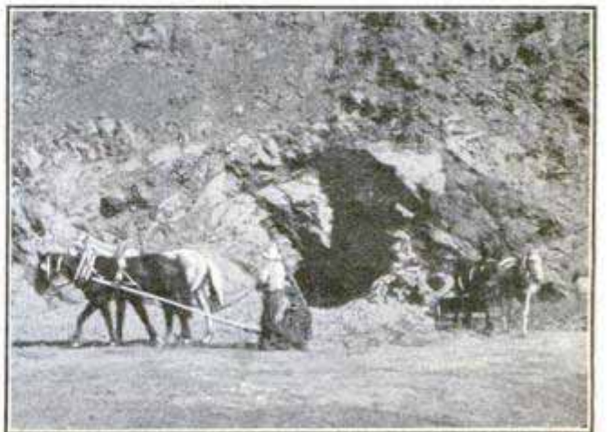
Opening of 100-Foot Tunnel into Mountain
