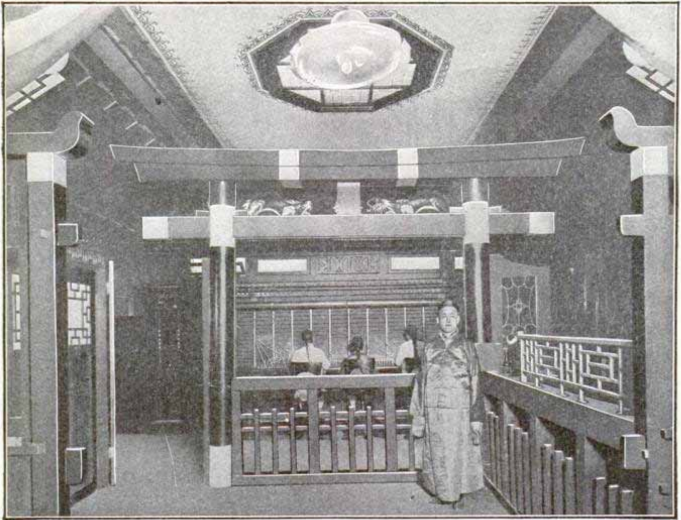
Interior View of Chinatown Exchange, Showing Manager and Operators at Switchboard
