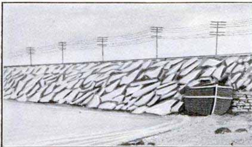
Covered with Sand and Rock to Form Part of Railroad Embankment
