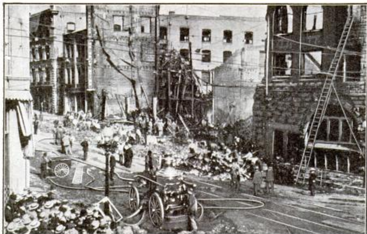
Broadway Side of The Los Angeles Times Building after the Explosion and Fire
