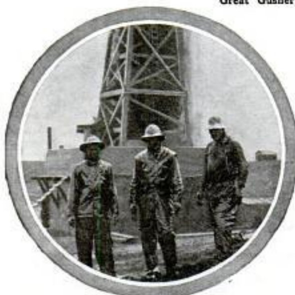
Engineer and Assistants at the Lakeview Gusher
