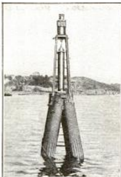
Pile Beacon Acetone Light—Will Burn Three Months at Cost of Two Cents per Day
