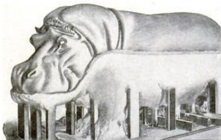
Making Plaster Mold of Sculptured Form
