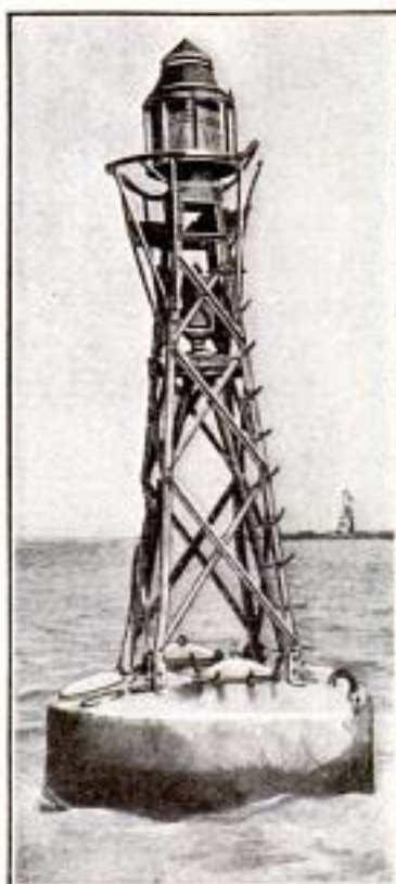
An Acetylene Beacon Buoy Which Has Been in Two Collisions with Ocean Liners near Greenville Pier, New York Harbor. Although Dragged Under Vessels' Bottoms, no Damage Was Done to Either Lighting or Whistling Functions
