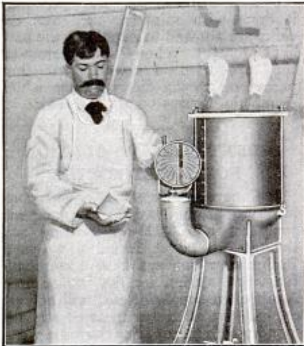
Automatic Scales Gives Customer Exact Amount of Lard Ordered
