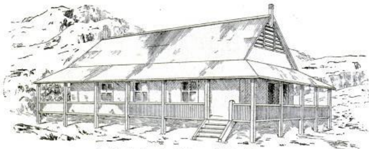
Porch Breaks Severity of Lines on this Iron House
