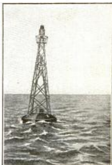
Wilson Combination Gas and Whistling Buoy, Lightship Type—Emits Powerful Blasts
