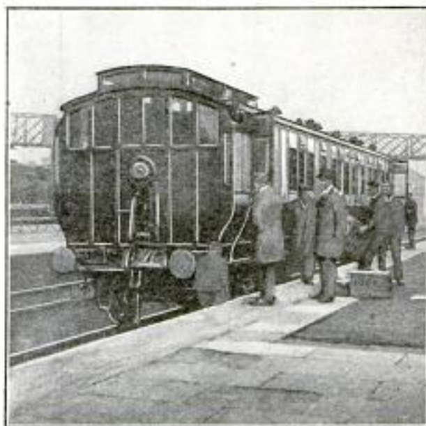
Slip Coach Brought to a Stop at Station
