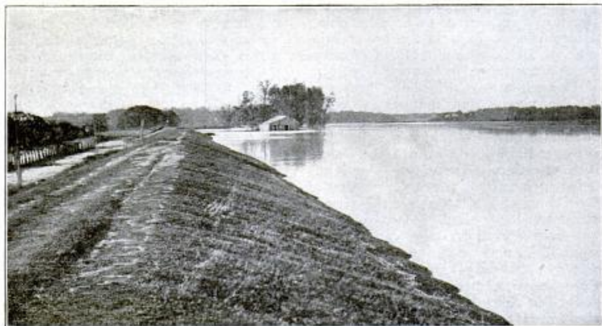
A View of a Levee Along the Mississippi
