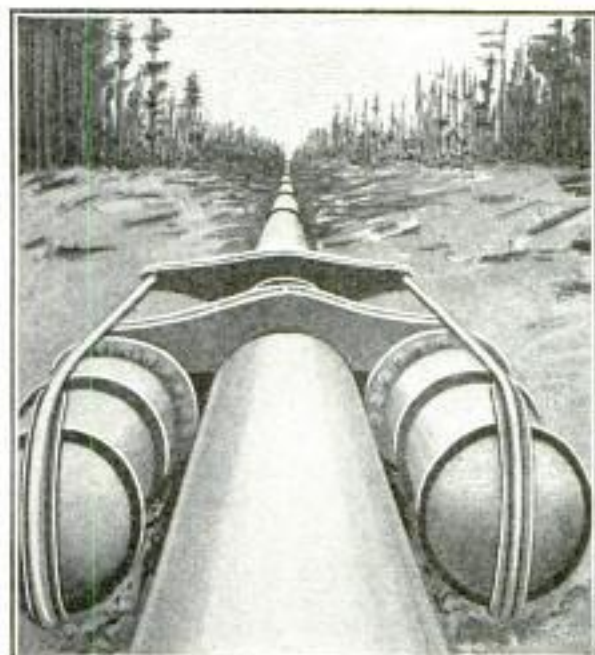
Expansion Safety Joints
