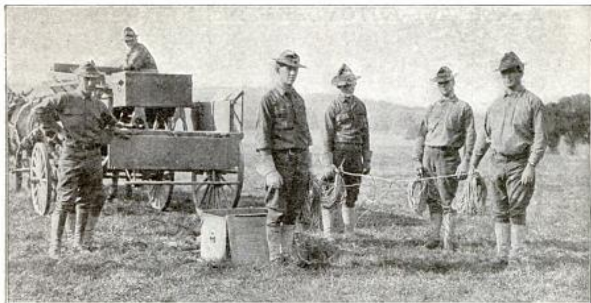
Insulated Wire Counterpoise Rolled Up
