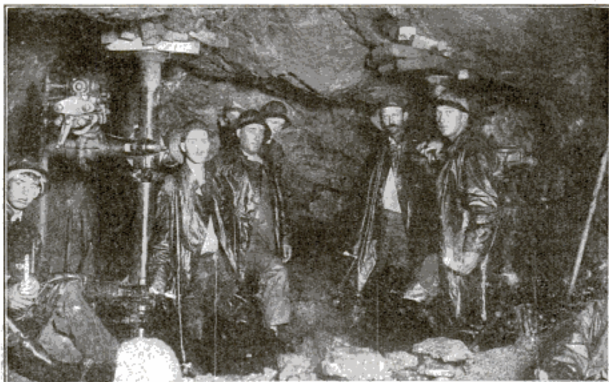
Scene in Gunnison Tunnel at Spot Where Accident Occurred—Photograph Taken a Few Hours Before Charge Was Placed
