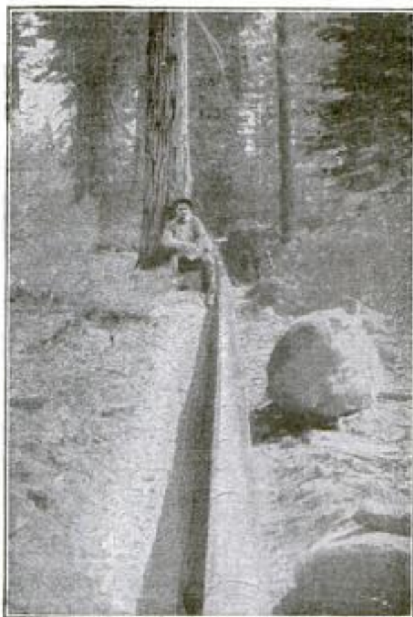
Pipe Line Down Mountain Side
