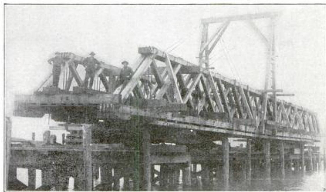
Raising the Bridge from Its Pier—The Bridge on Scows—Loaded on Cars
