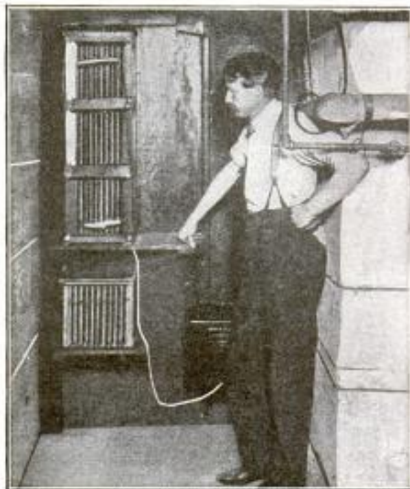
Ozone Generator in Chicago Library
