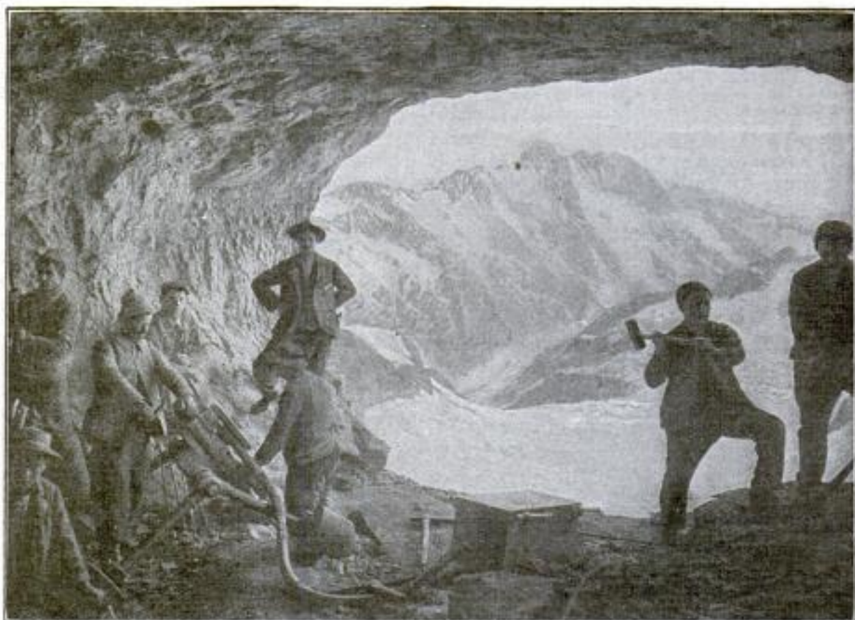
Working an Electric Drill at a Height of 10,000 Feet
