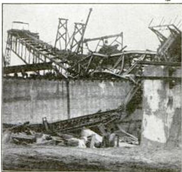
Damage Ascribed to Labor Troubles
