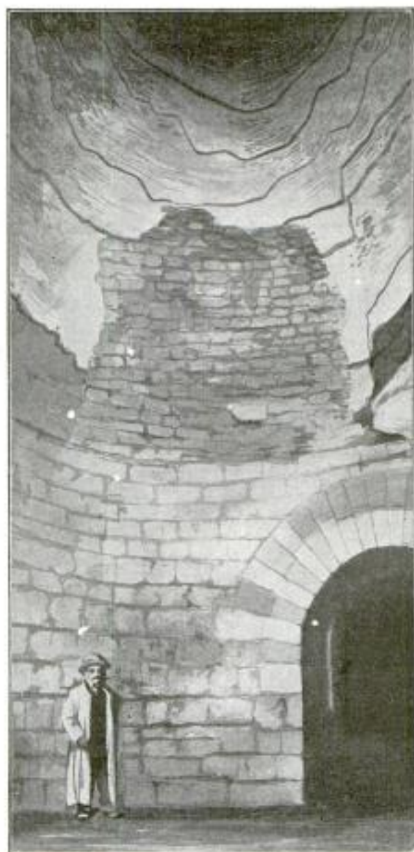
Quarry Forming Domed Chamber
