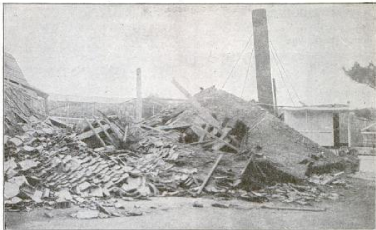
A Ruined Warehouse
