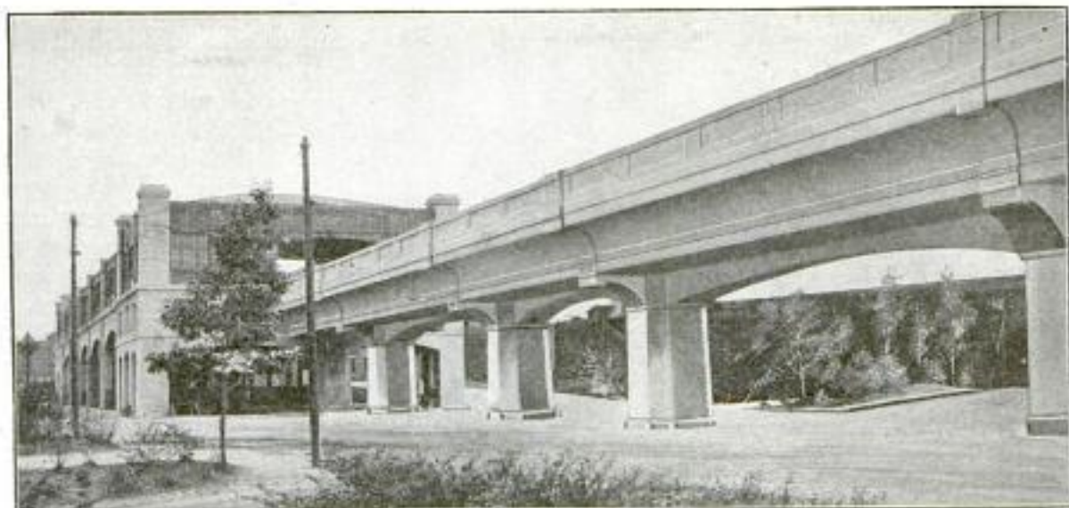
The Handsome Elevated Roadway After Embellishment with Concrete
