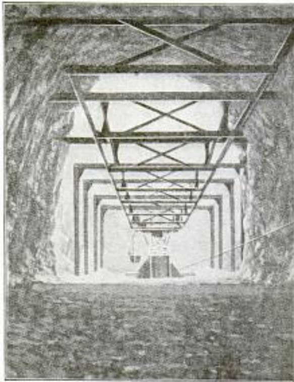
Rails Take Place of Cables in Tunnel
