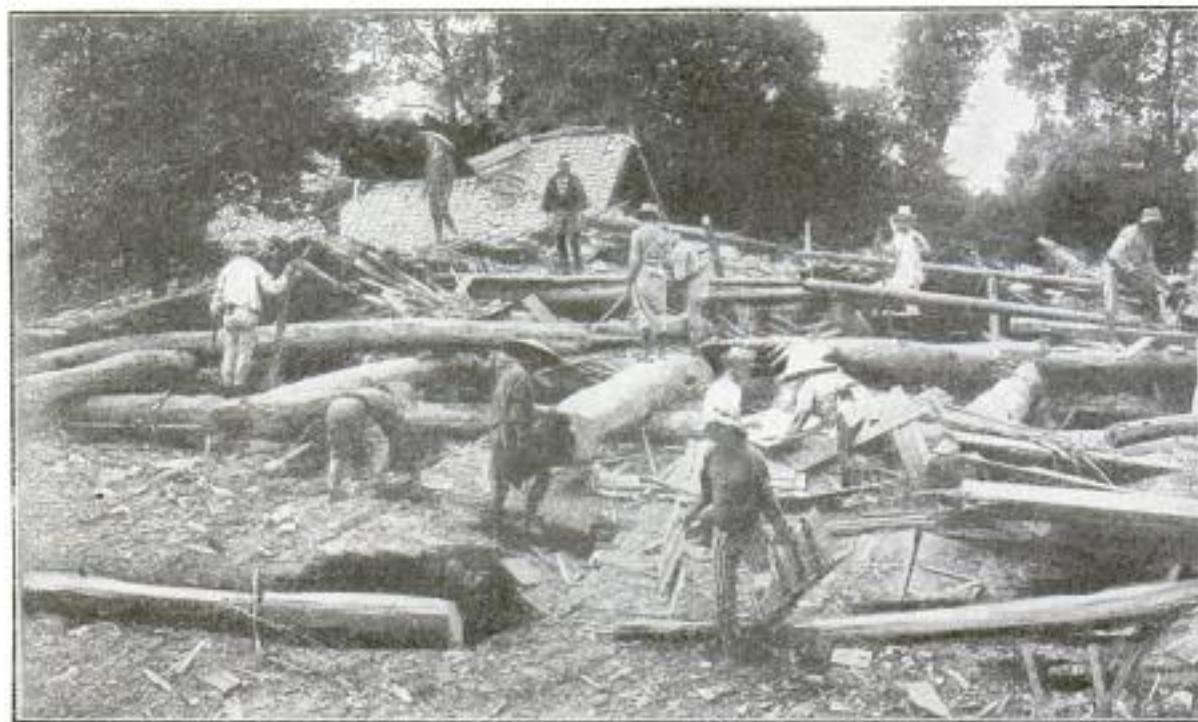
Clearing Away Wreckage
