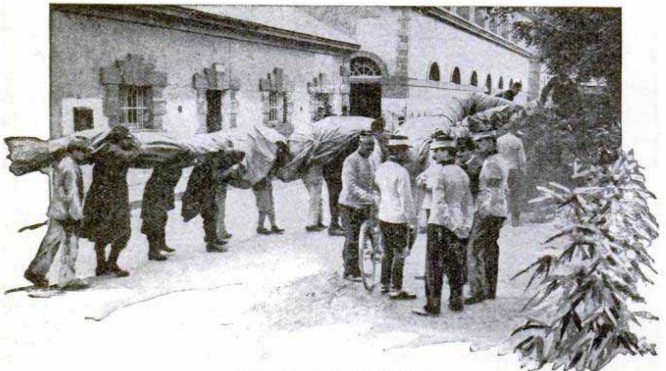
Removing the Torn Gas Envelope
