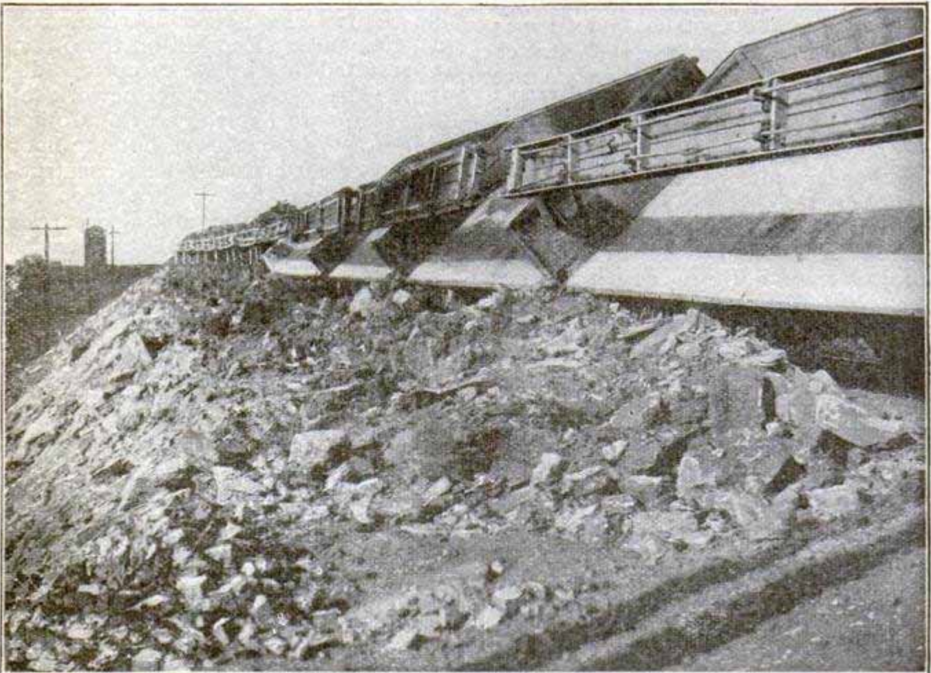
Dumping a 2,000,000-Ton Hill into a Hollow 3 Miles Distant—Dumping a Train of Cars by Compressed Air in Three Minutes
