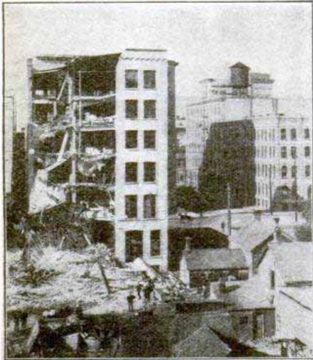
Result of Water Tank's Fall
