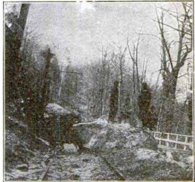
50-Ton Boulder Blocking Tracks—After It Was Blasted
