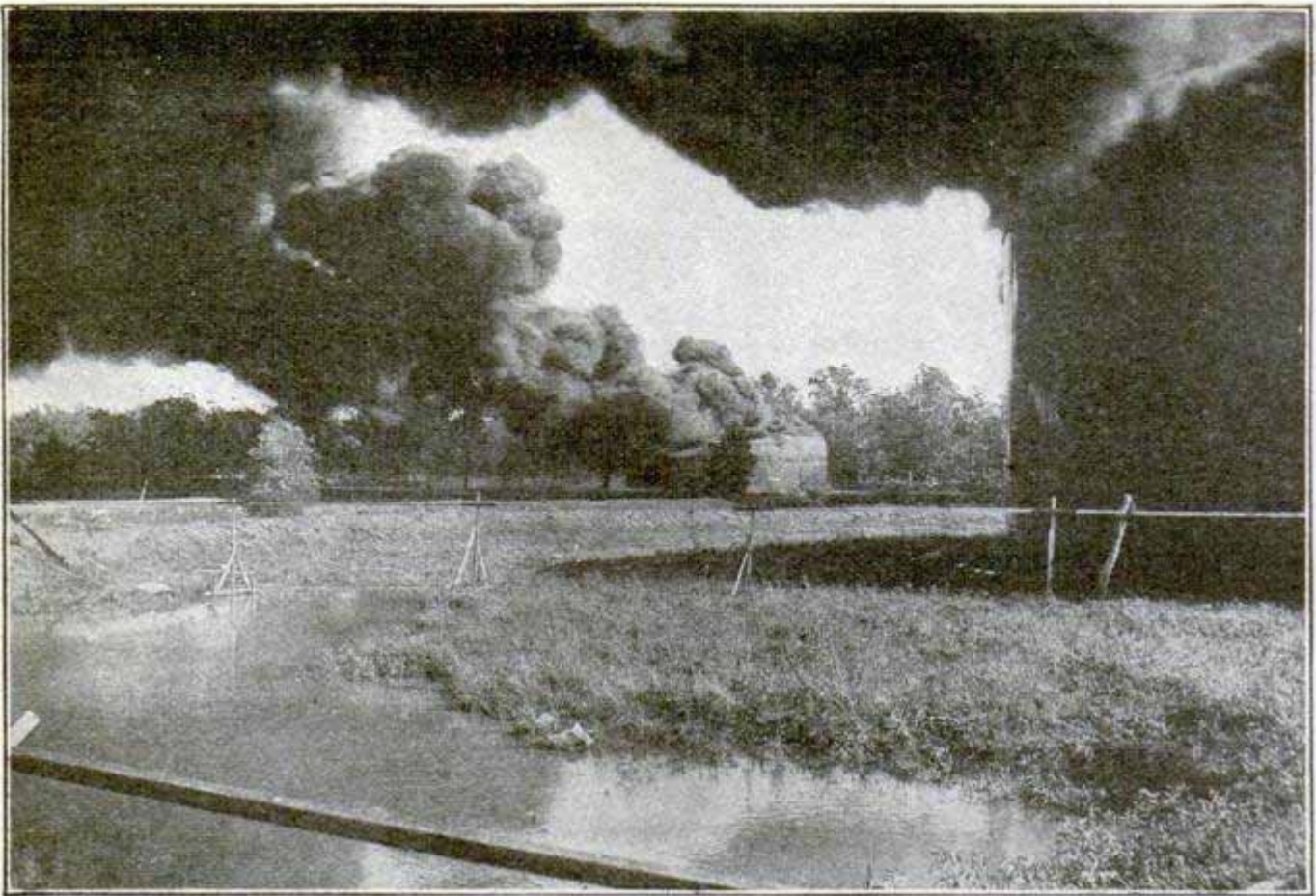
Oil Tanks Ignited by Lightning
