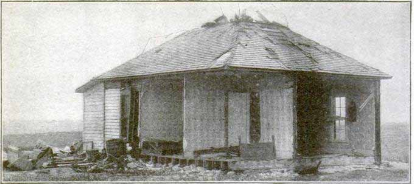
Farmhouse Damaged by Storm
