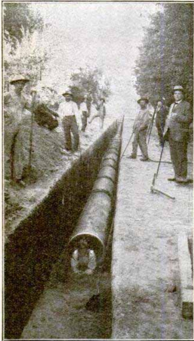
Laying Stave Pipe in Street
