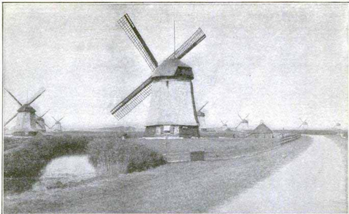
Windmills for Water Drainage, Amsterdam, Holland—16 Mills Working Always Together
