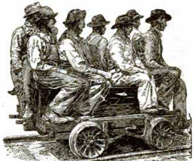
Motor Section Car Carrying Nine Men and Tools
