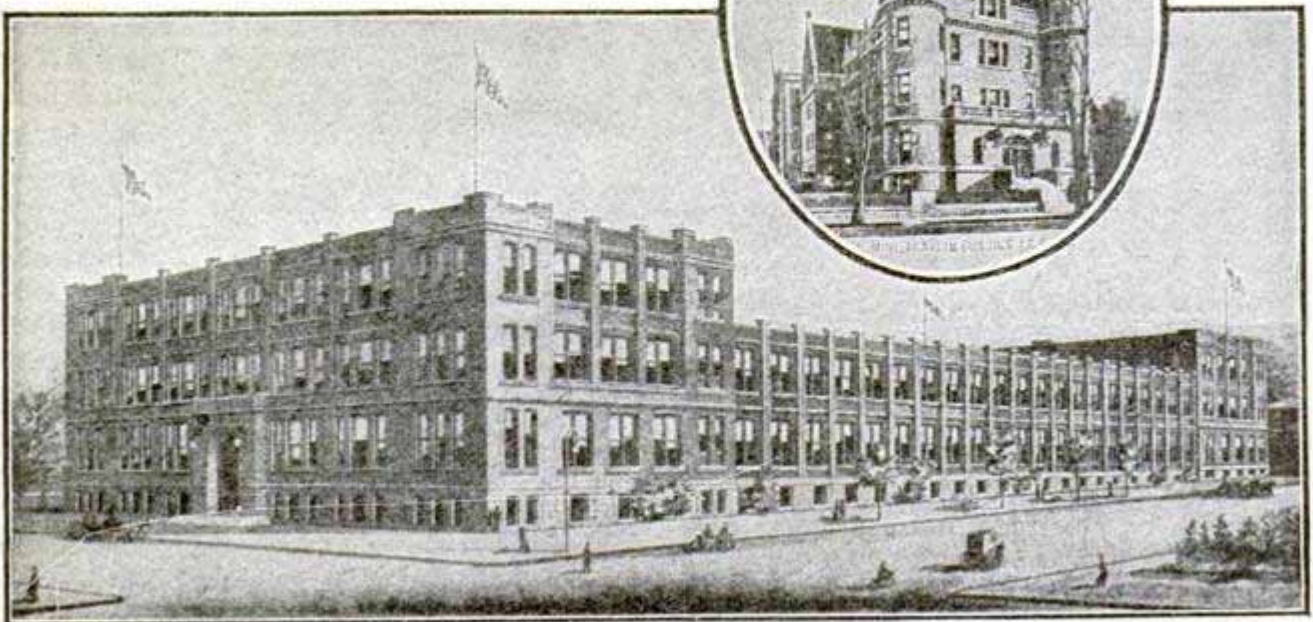
I. C. S. BUILDING OCCUPIED ENTIRELY BY THE SCHOOLS
