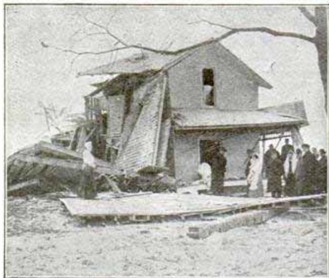
Completely Wrecked by Acetylene Gas
