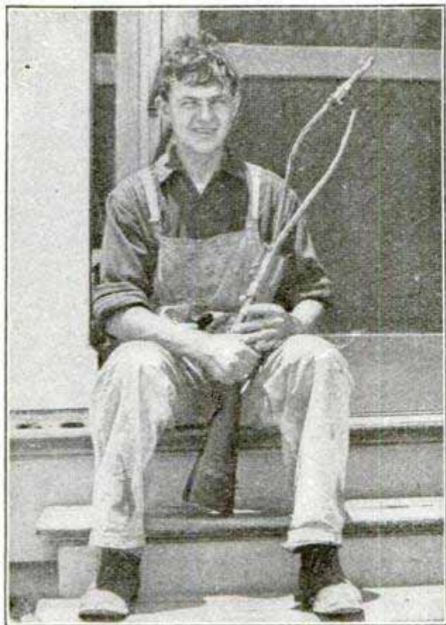
Clogged Rifle Split by Discharge
