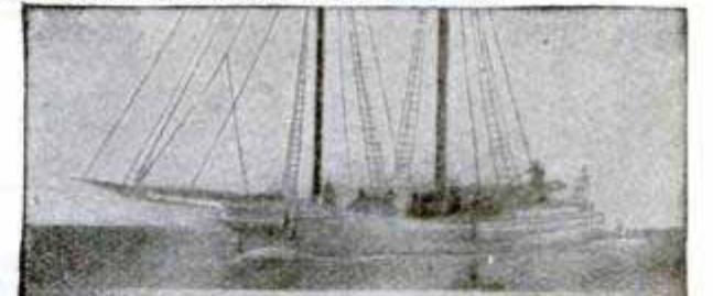
POWER —Capt. Norman Evans, of Millville, N.J., pushing schooner 53 ft. long, 16 1/2 ft. beam, with his 2-cyl., 12 H.P. motor boat.
