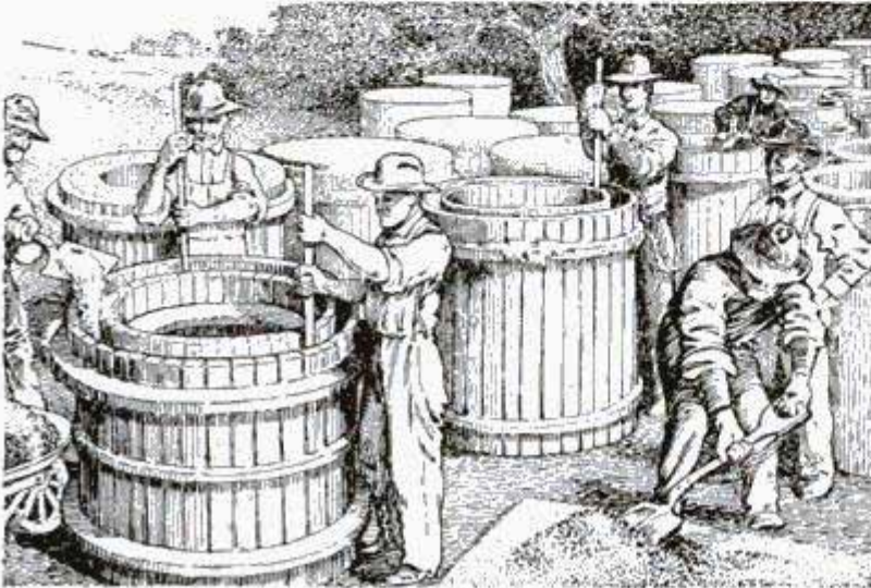
A Stock of Concrete Pipe Moulds in Which Pipe Is Made
