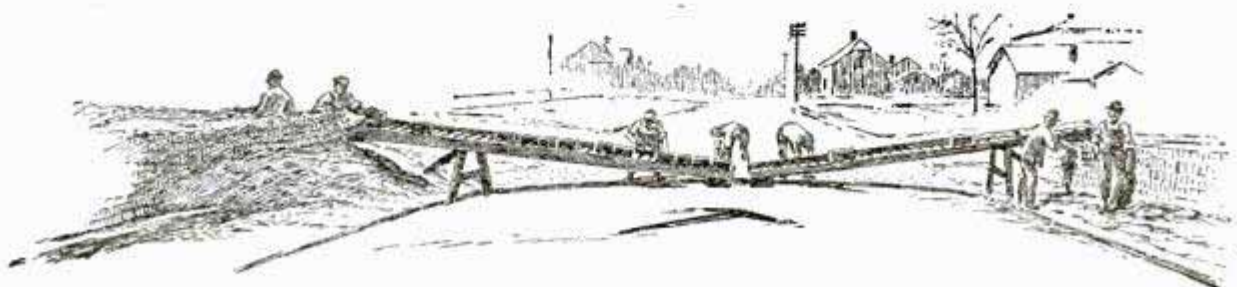
Chutes Facilitate Handling Brick
