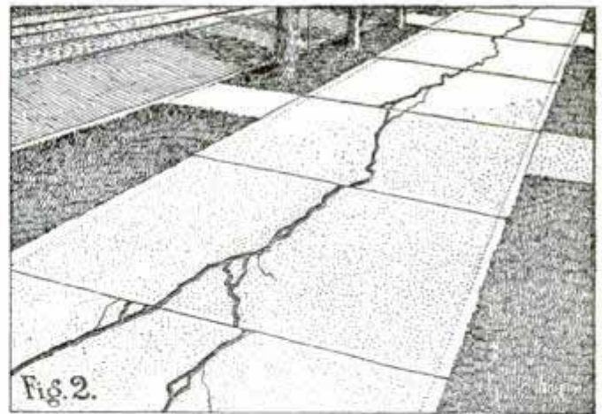
Longitudinal Crack through Center
