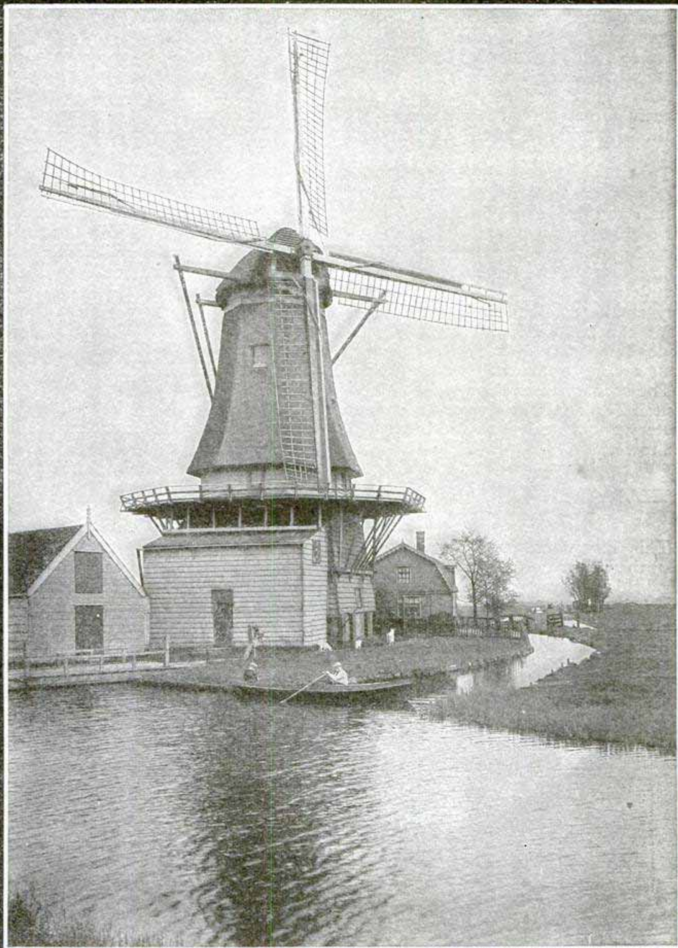
Windmill in Holland Furnishing Power to Wood-Working Shop in Lower Part of Building
