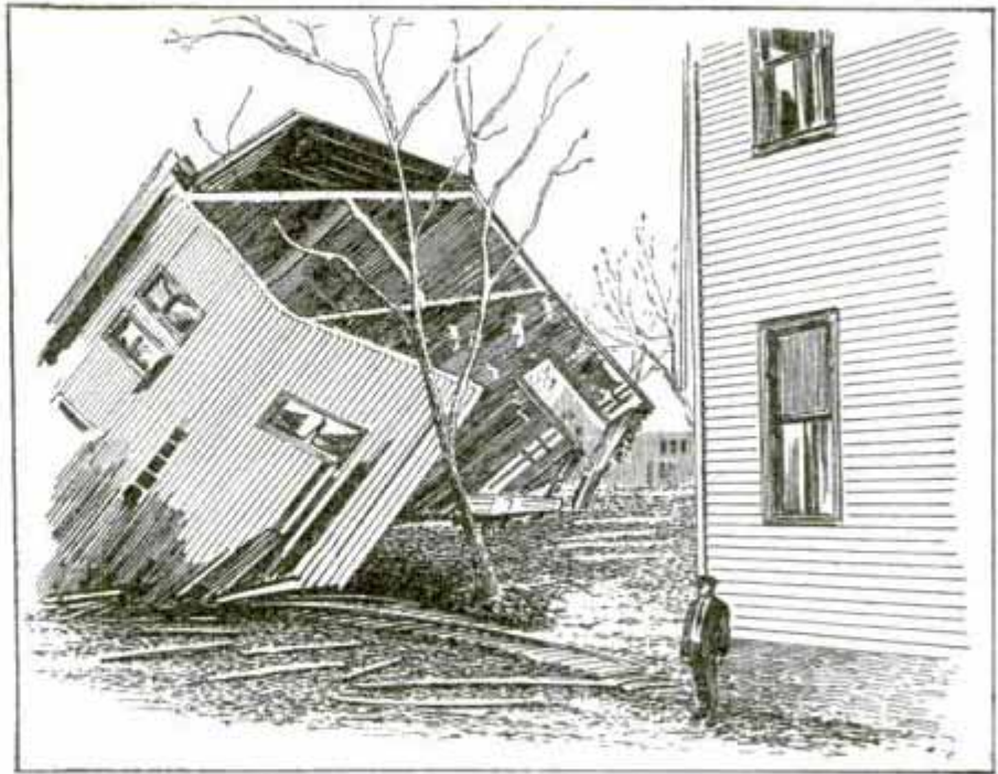
Storm Cut House into Two Sections
