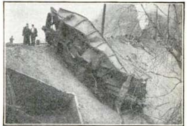
On the Embankment—In the Valley Below— Wreck of a Steel Car
