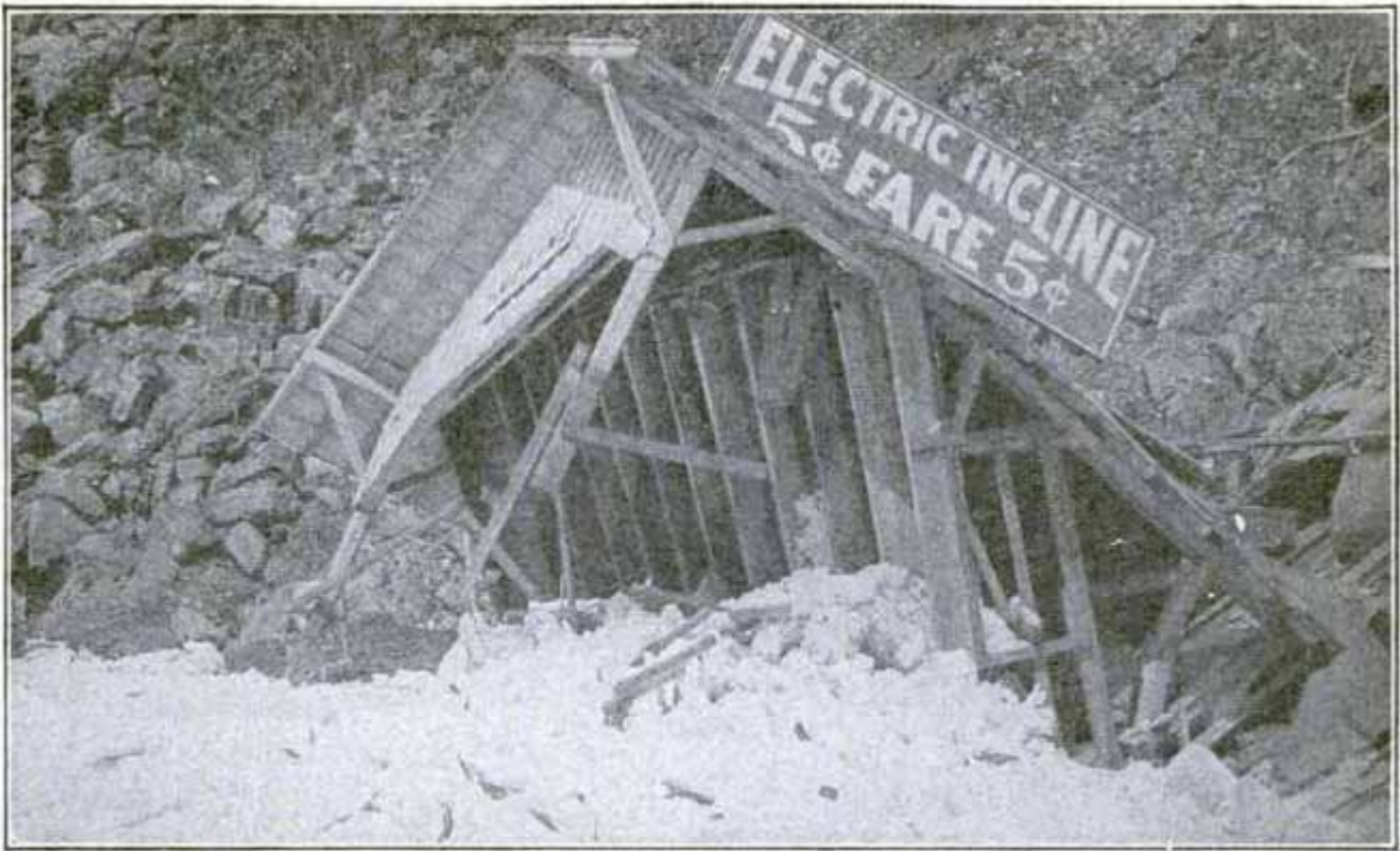
Fig. 5—Wreck of Incline Railway
