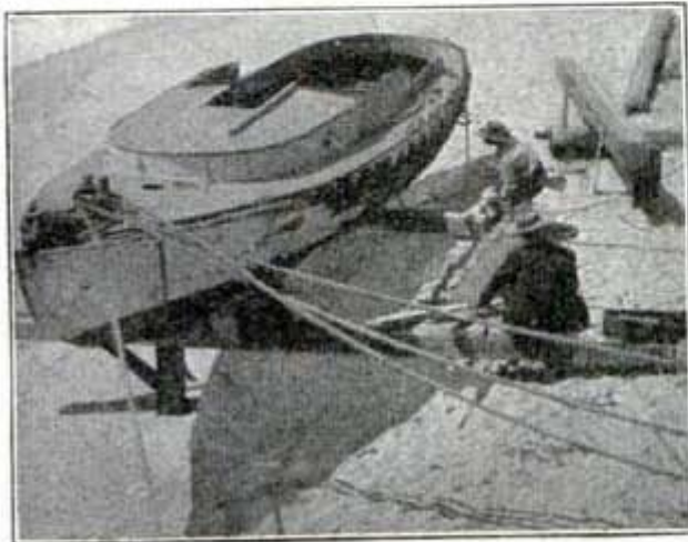
Emergency Ship Yard
