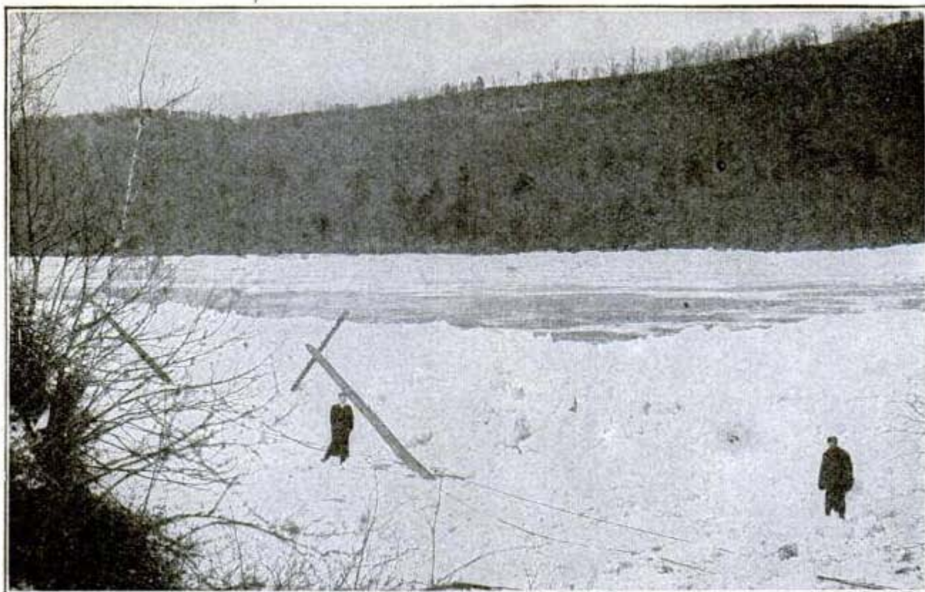
Fig. 12—Trolley Line Under 25 Ft. of Ice at This Point
