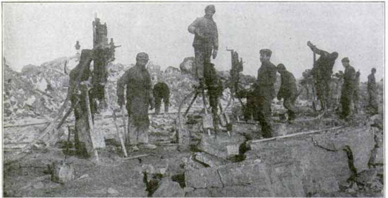
Pneumatic Drills Preparing the Way for the Blasts
