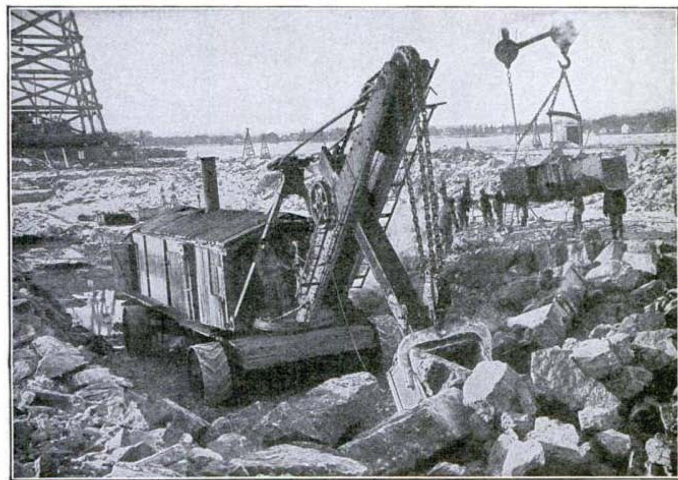
First Gash in River Bed and the Conveyer—Great Steam Shovel Gathering Up the Shattered Rock
