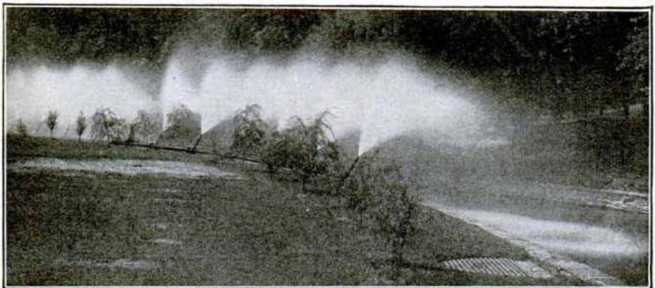
The Water Is Sprayed to Cool It
