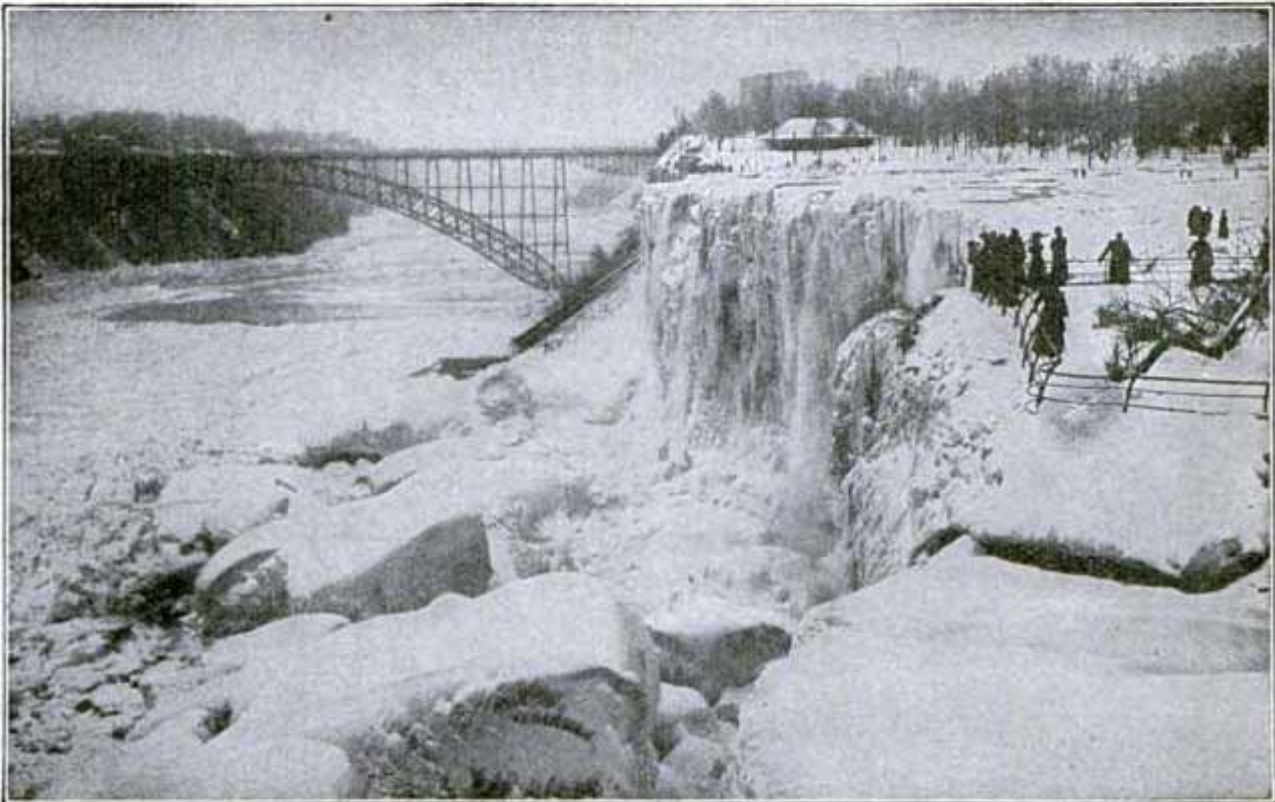
Appearance of American Falls During the Jam
