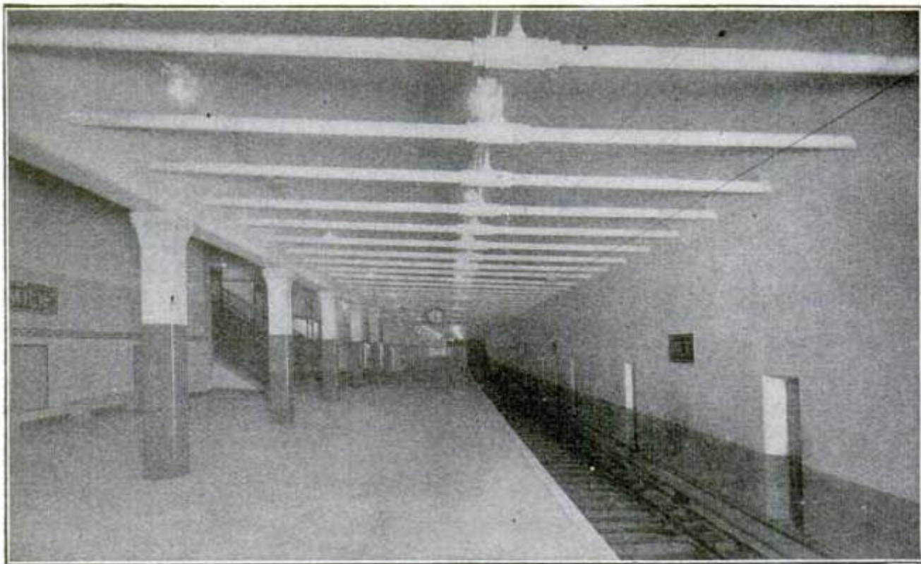
One of the 350-Ft. Platforms
