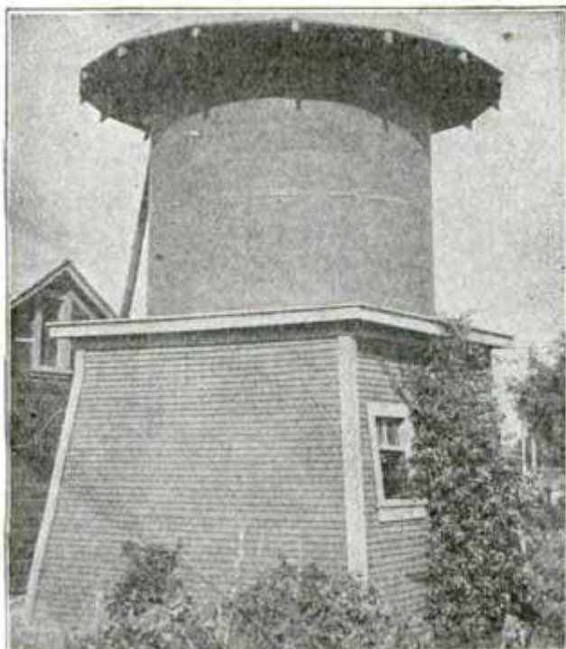
A Water Tank of Galvanized Iron
