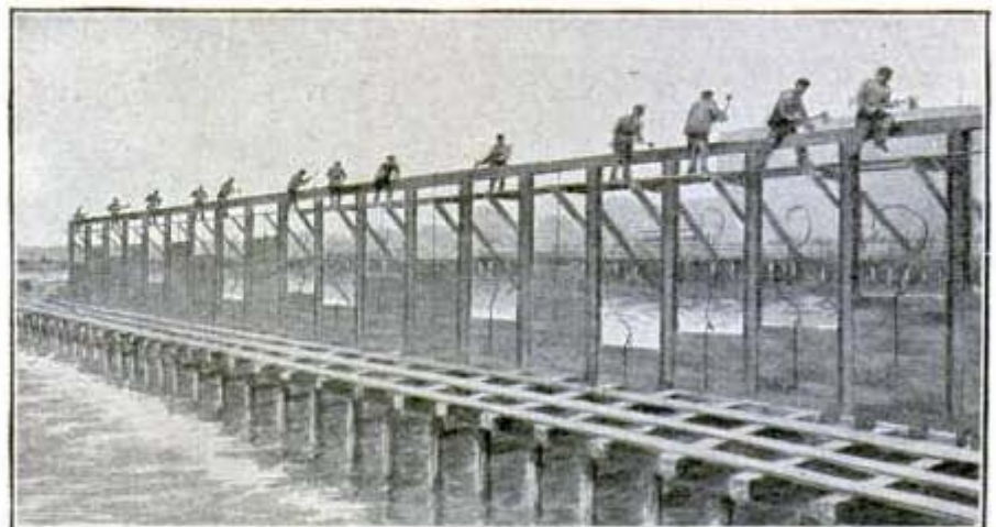
Releasing the Gates of the Shut-Off Dam Which Stopped the Tidal Flow of the River Basin
