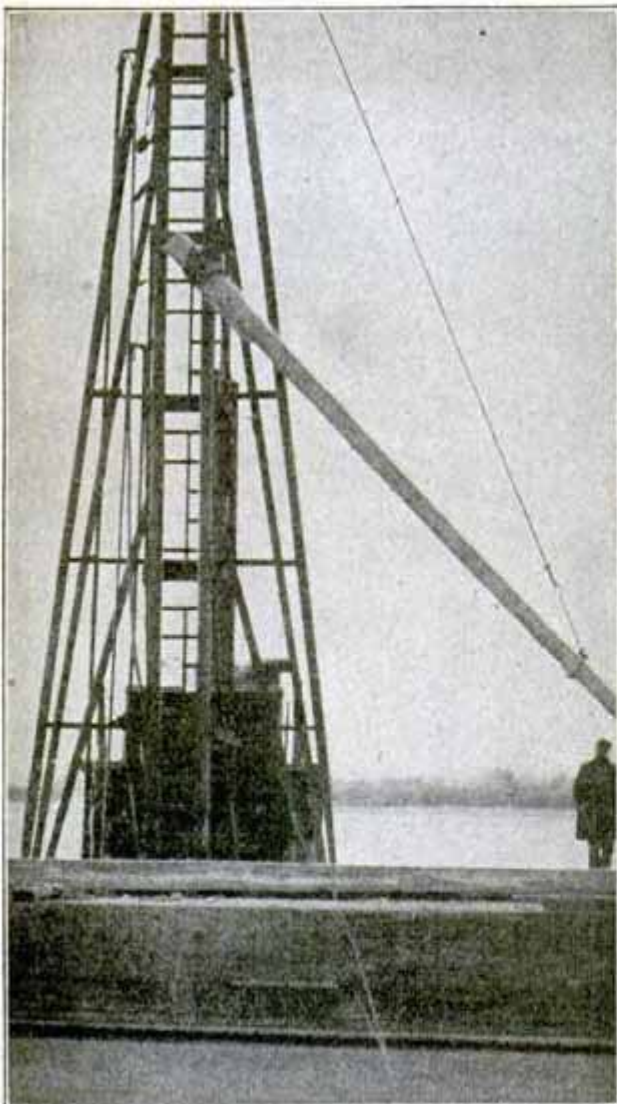
Sinking Concrete Piles
