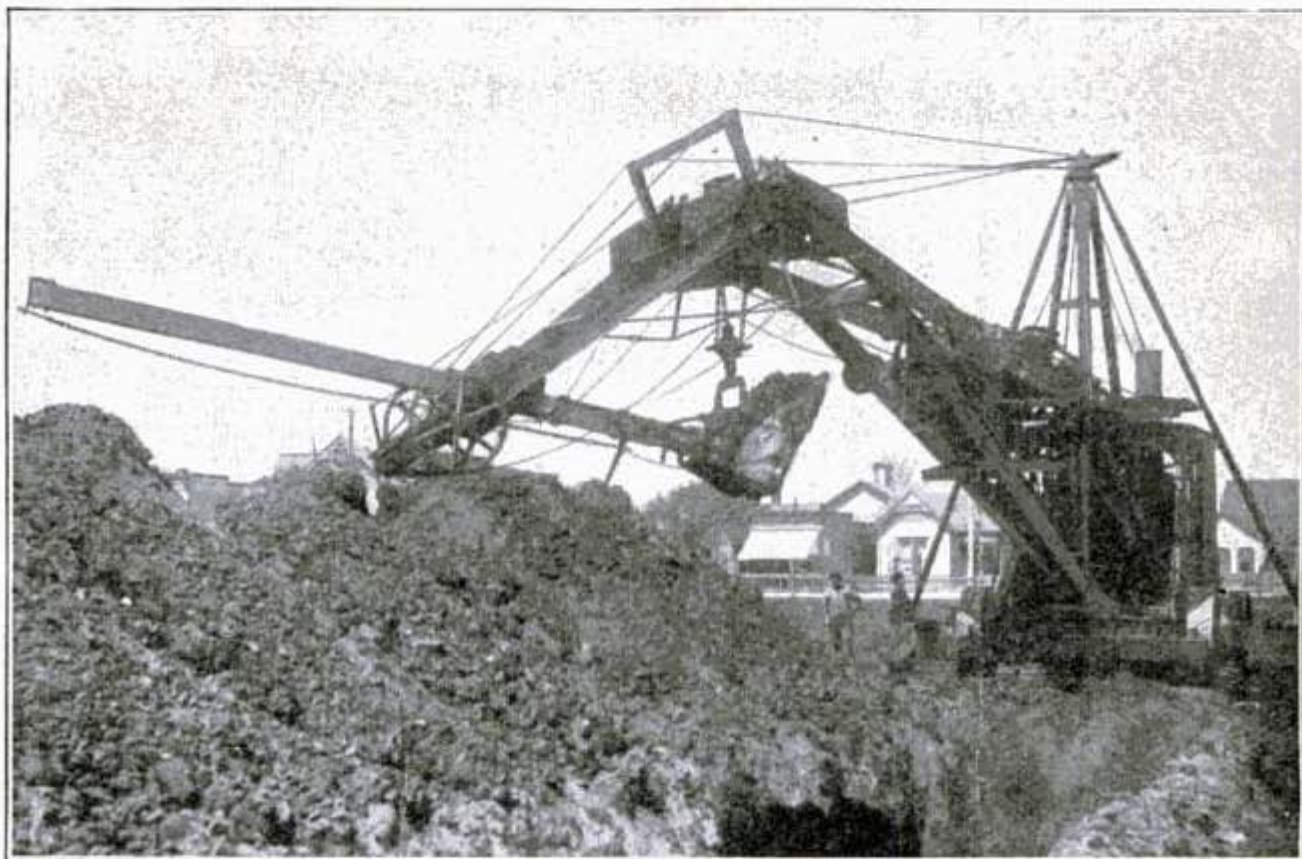
Machine Digs Trench 10 Ft. Wide and 18 Ft. Deep
