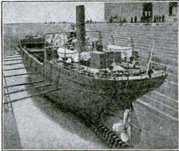
"Transporter" Being Submerged to Receive Submarines
