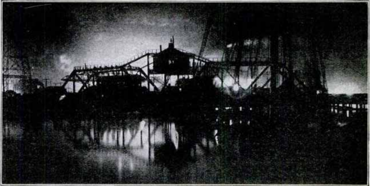
Taken at 10 O'Clock at Night
