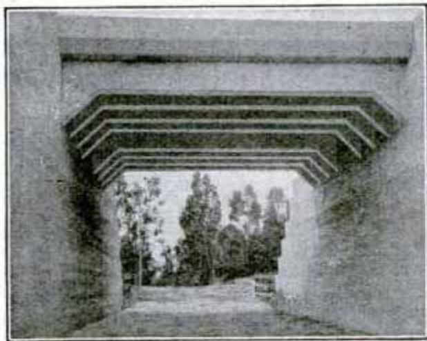
Unique View of Bridge
