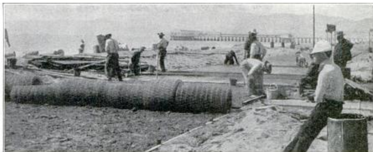
Building the Mile-Long Sidewalk
