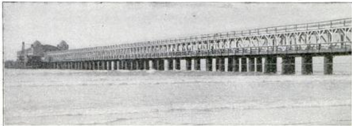
New Method of Constructing Pier Supports
