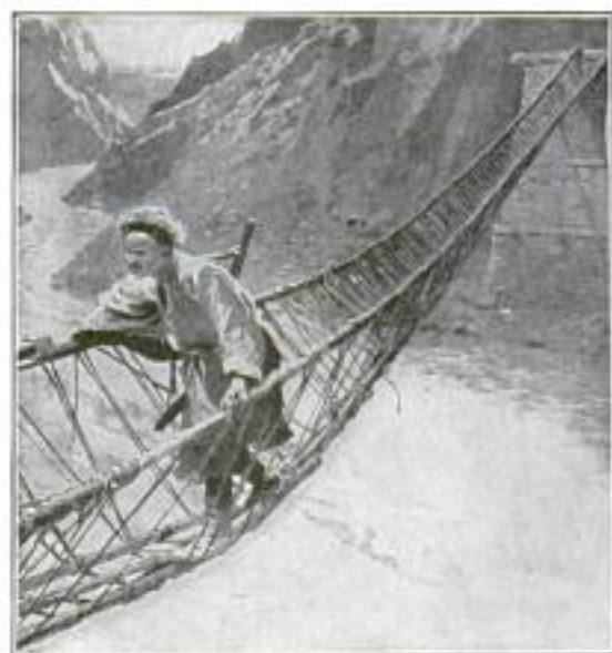
In Hindustan, near the Indian frontier, the country is rugged and improvements are of a very primitive though often ingenious character. The illustration shows a suspension bridge built by the natives by splicing bamboo. The construction closely resembles the inverted frame of a dirigible airship.—Courtesy London Graphic.
