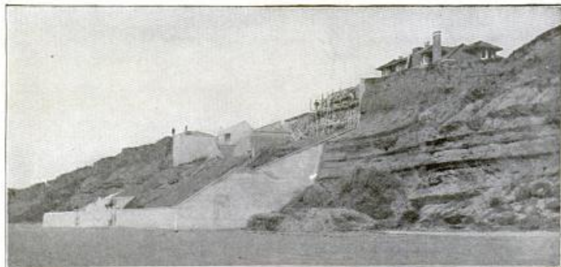
The Concrete Wall Along the 60-Ft. Bluff
