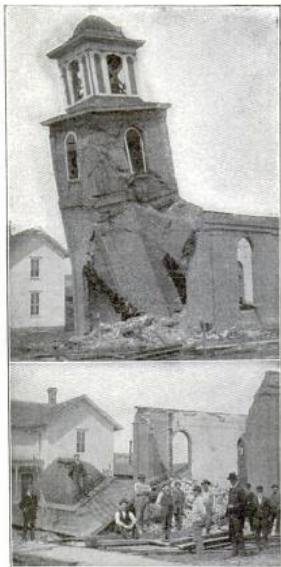
PICTURE OF FALLING CHURCH TOWER
