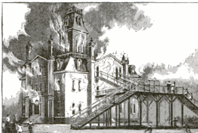
Safety Stairs 35 Ft. from Building
