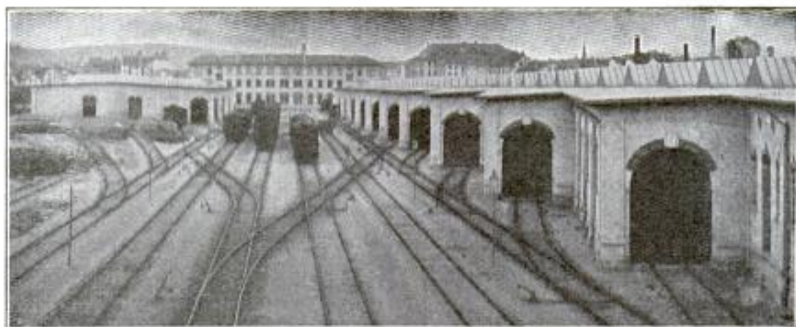
Standard Type of English Freight Houses Permitting of Largest Possible Number of Switch Tracks into the Building
