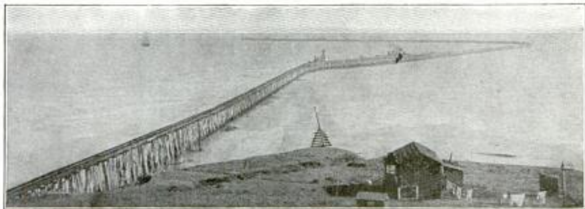
This Breakwater Extends Two Miles Out Into the Sea
