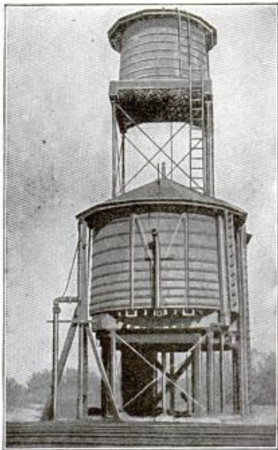
High Tank for Fire Pressure
