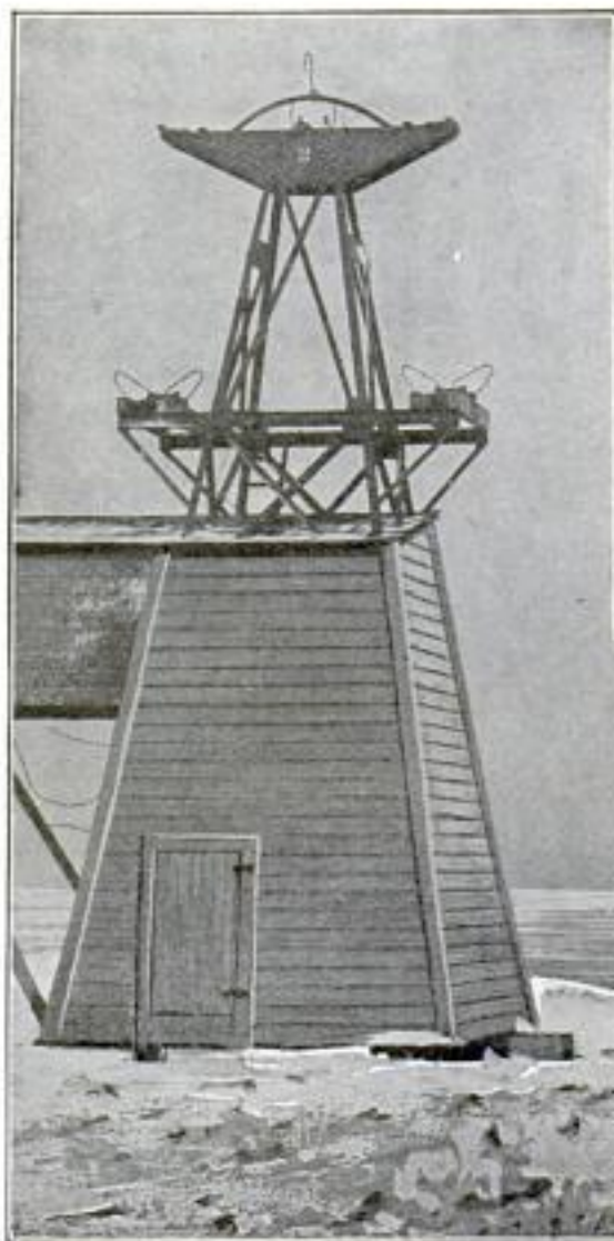
Remaining Towers of the Wrecked Aerial Railway
