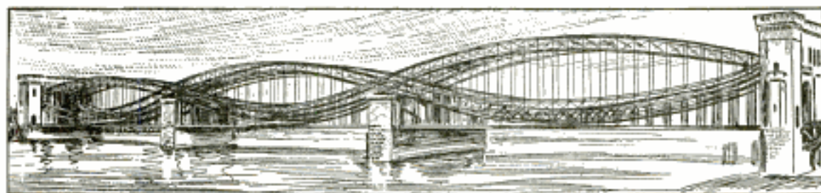
Elbe Bridge Near Hamburg—Each Span 325 Ft. Long
