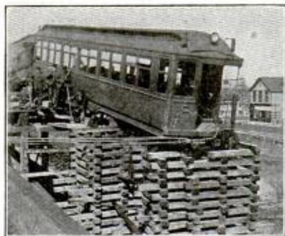
Crib Work to Raise Car
