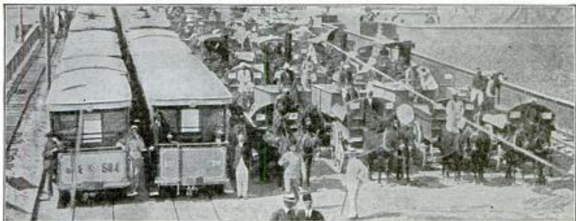
After three years of work, the largest bridge across the Nile has just been completed from Cairo to the island of Rodah. The bridge is 1,740 ft. long, and 65 ft. wide. The official test subjected the bridge, span by span, to a weight equal to 400 lb. per square yard. To accomplish the test 20 cars, 24 water carts, and 20 dust carts, all of which were loaded with cement, sand and water, and 8 steam rollers stood on each span for 24 hours. The entire procession crossed the bridge from end to end.
