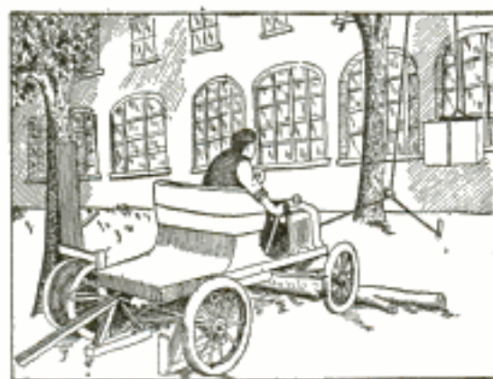
Hoisting with an Auto
