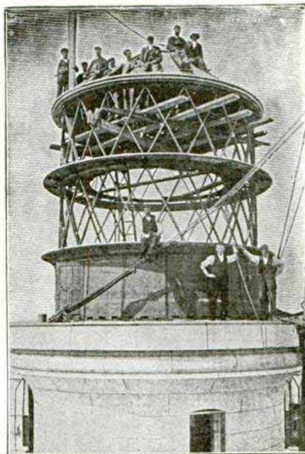
Lantern in Course of Erection
