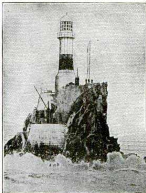
Fastnet Rock. Showing Old Lighthouse and New Tower Under Construction
