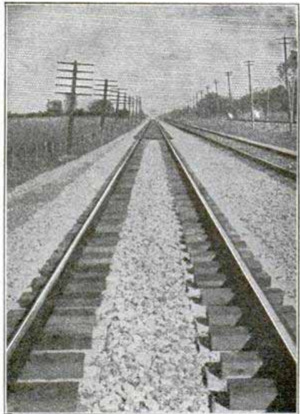
"A 'Tie' Consists of Two Blocks of Concrete"
