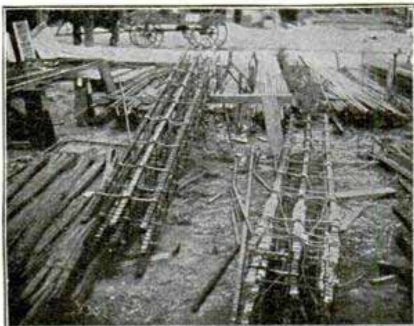
Steel Reinforcements for Concrete Columns
