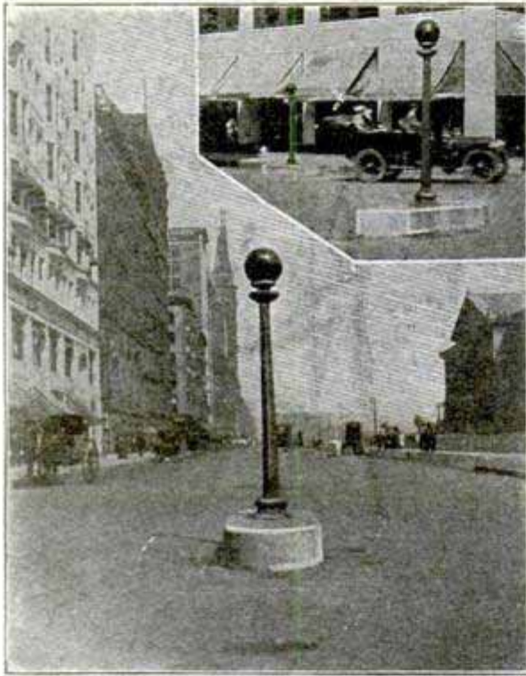
Danger Sign in Street
