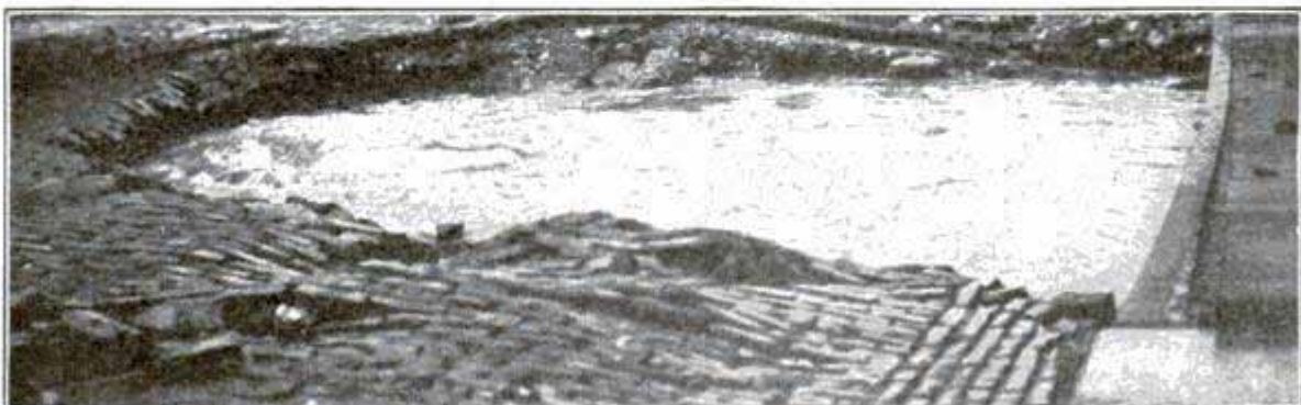
Condition of Street after Break Was Controlled
