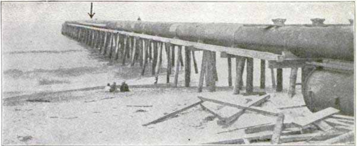
Arrow Shows where the Pipe Collapsed
