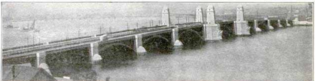
New $3,000,000 Bridge over Charles River
