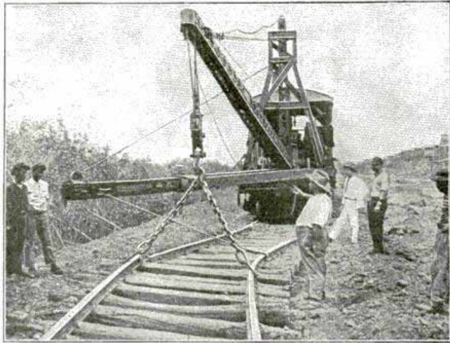
Moved 6000 Ft. of Track 4 Ft. Sideways in 8 Hours
