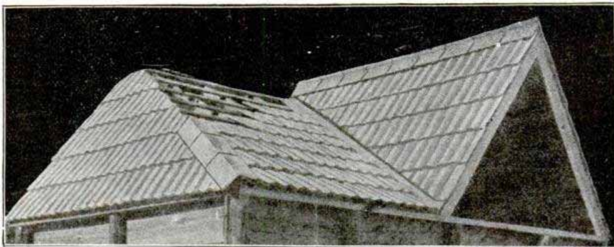
Tinted Shingles Are Now Made of Cement
