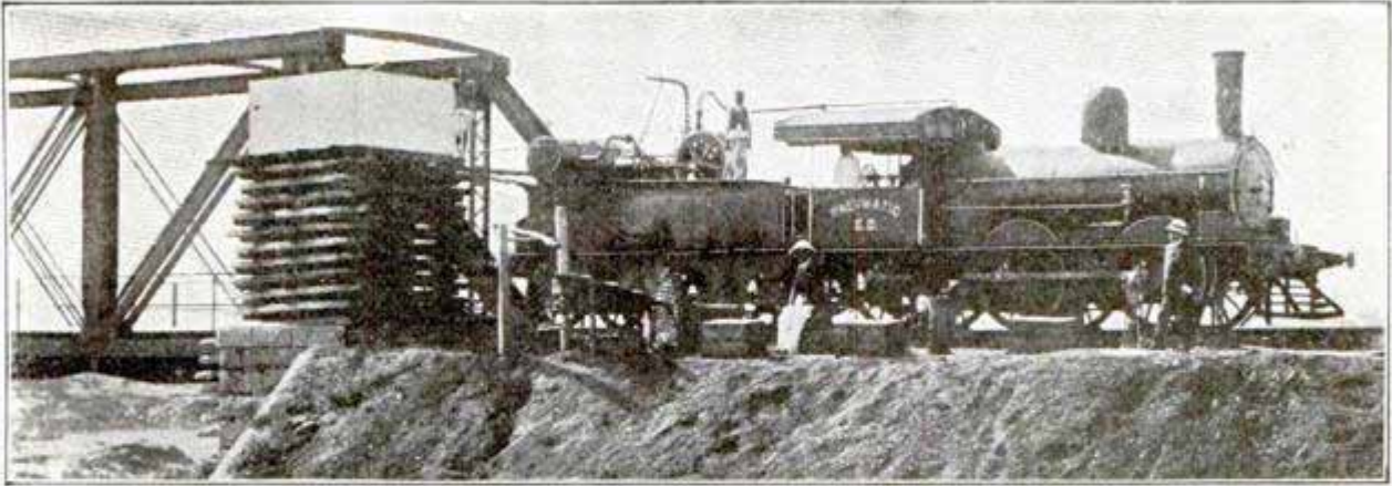
Compressed Air Plant for Working Pneumatic Tools on Indian Locomotive
