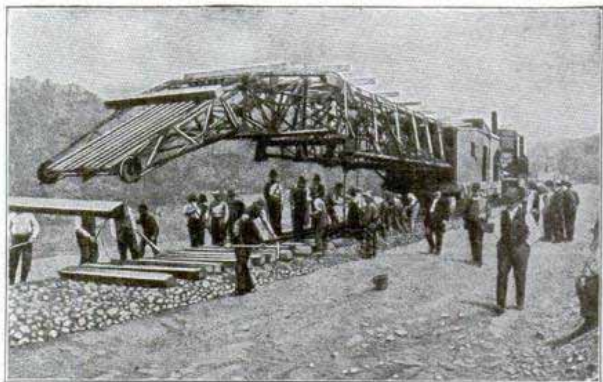
Track Laying Machine
