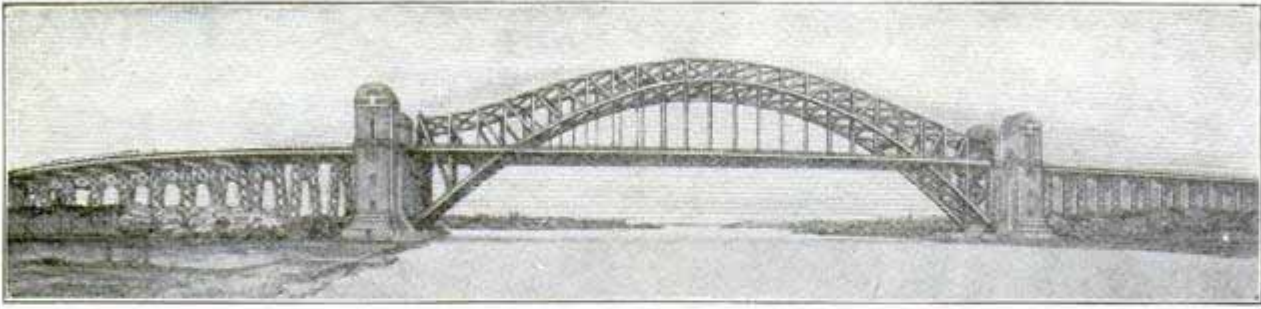
This Will Be the Largest Steel Bridge in the World
