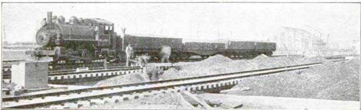
Piles Will Be Leveled; then Submerged
