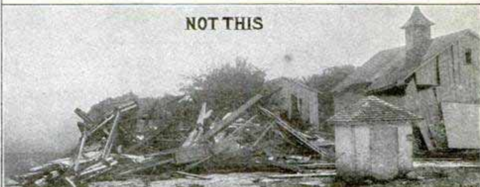
From a photograph showing wreck caused by collapse of old-fashioned elevated tank.
