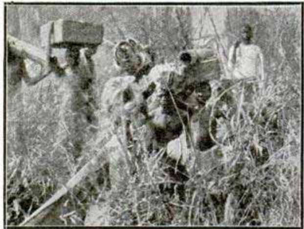
Building the Line
