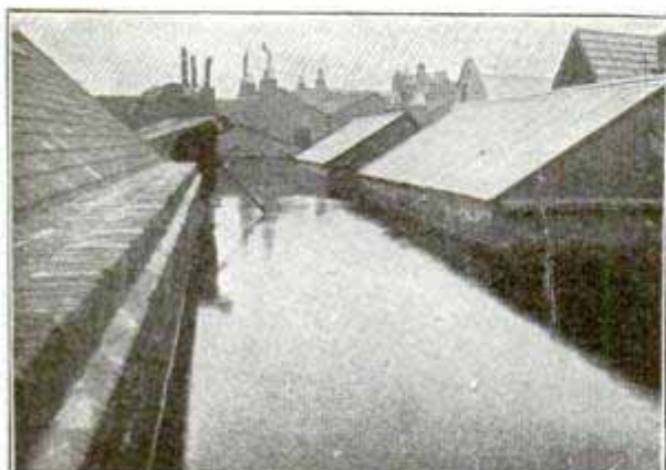
Huge Tank on Roof
