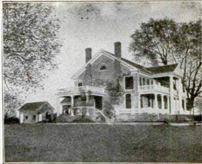
Residence of W. T. Ashford, Atlanta, Ga. Supplied by Kewanee Water System
