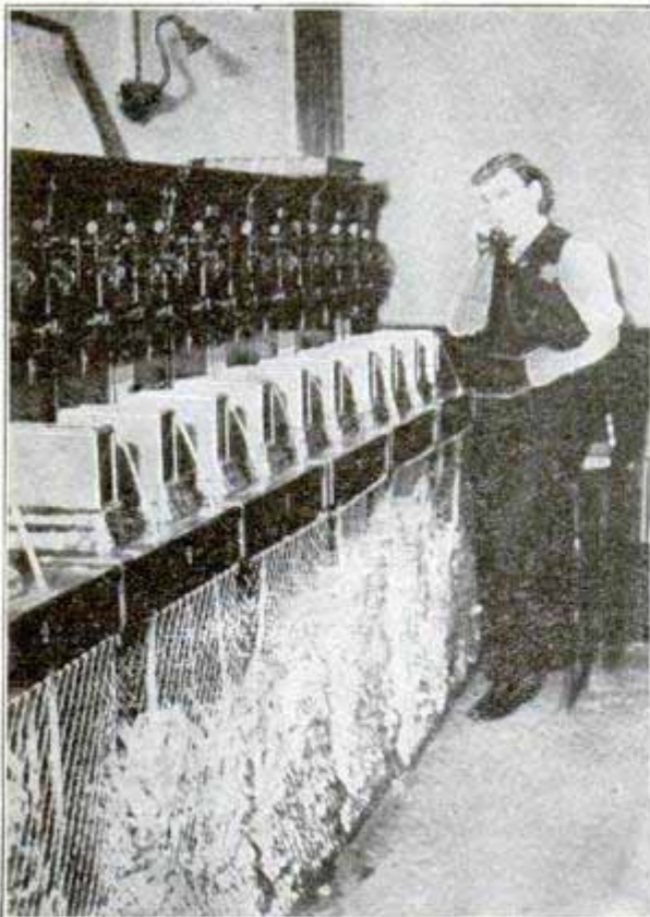
Switchboard at Central Office
