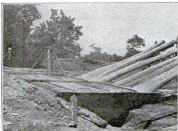
Treating Chestnut Poles by Tank Method
