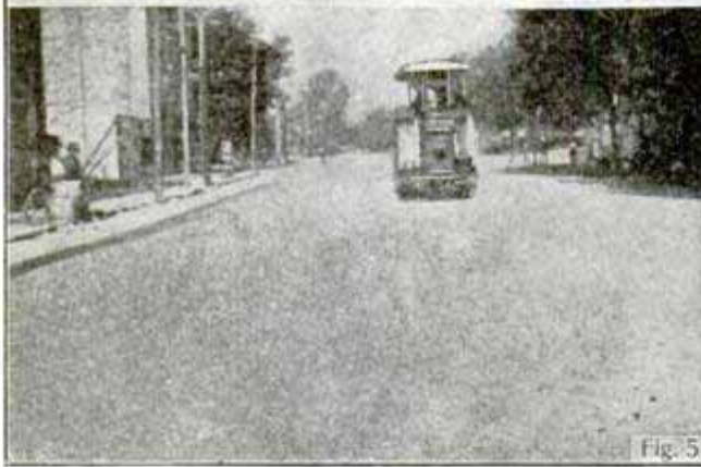
Fig. 1--Sweeper Cleaning Street. Fig. 2--Putting on the Tar With a Sprinkler. Fig. 3--Spreading Tar With Brooms. Fig. 4--Covering Tar With Finely Crushed Stone. Fig. 5--Finishing With Steam Roller. Fig. 6--The Completed Roadway.
