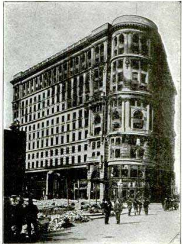
No. 4.--Flood Building--12 Stories--Interior Burned-- Can be Restored for $100,000
