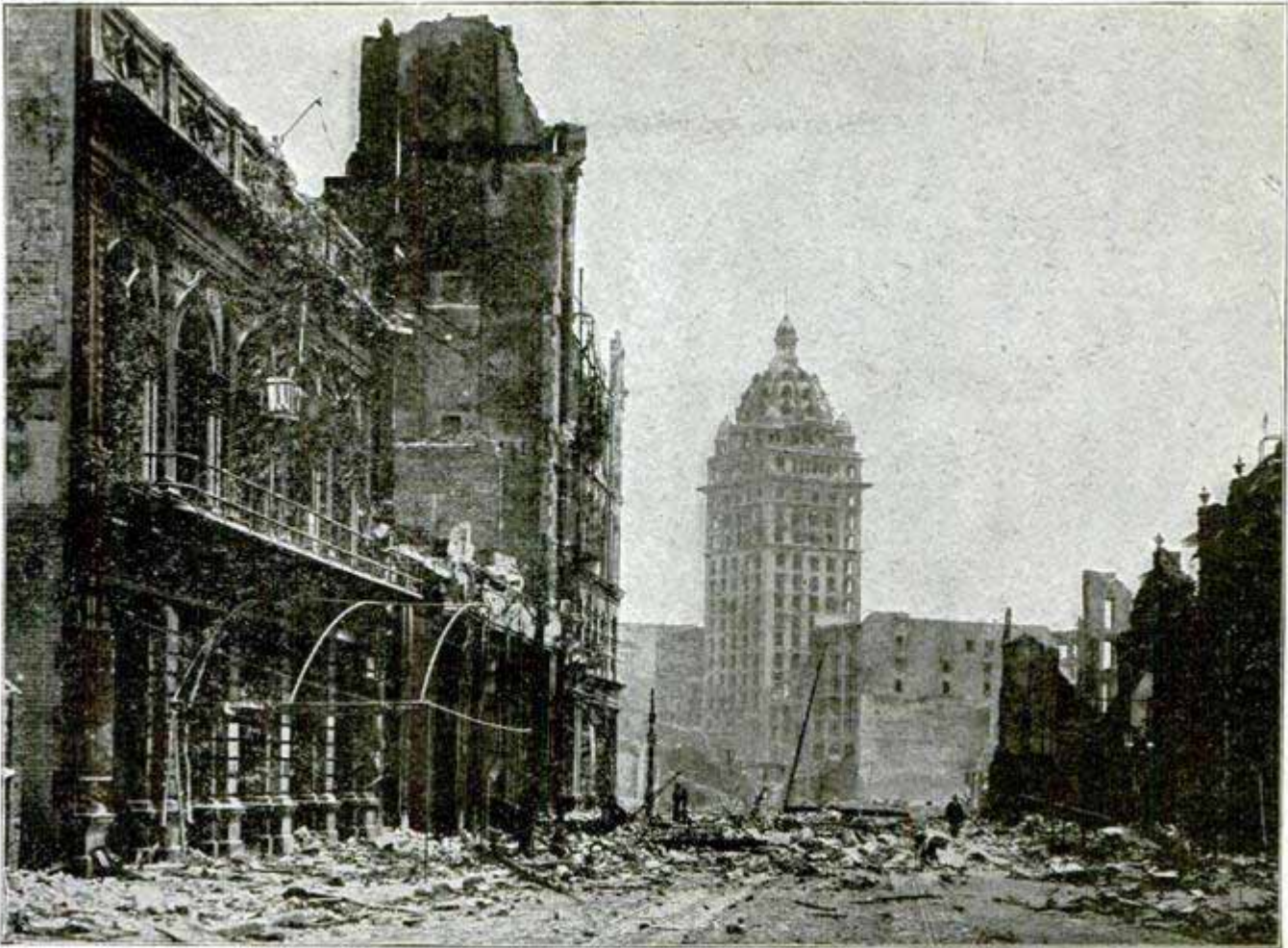
No. 3.--Call Building, 300 Ft. High--Interior Burned Out, but no Visible Cracks in Outer Walls
