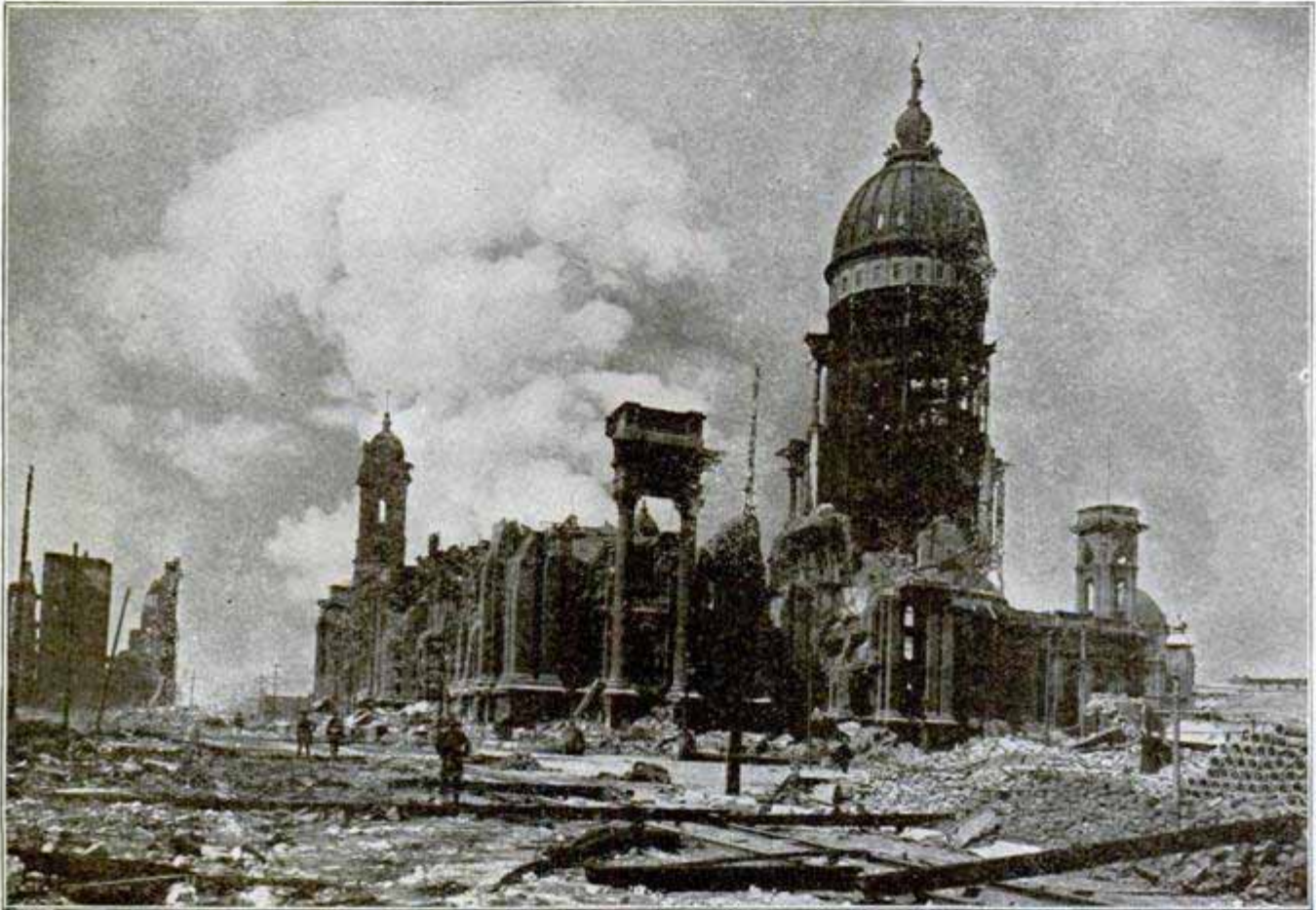
No. 1.--City and County Building: A Total Wreck
