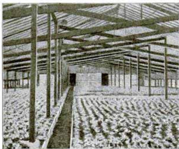
Interior of Glass-Covered House
