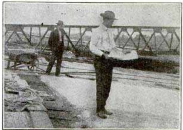
Laying the Concrete Roof
