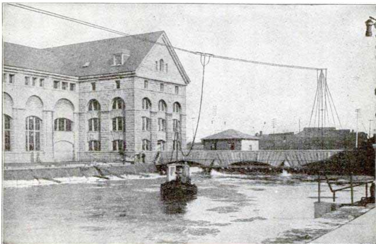
Trolley Boat to Disperse Floating Ice at Niagara Falls Power Plant
