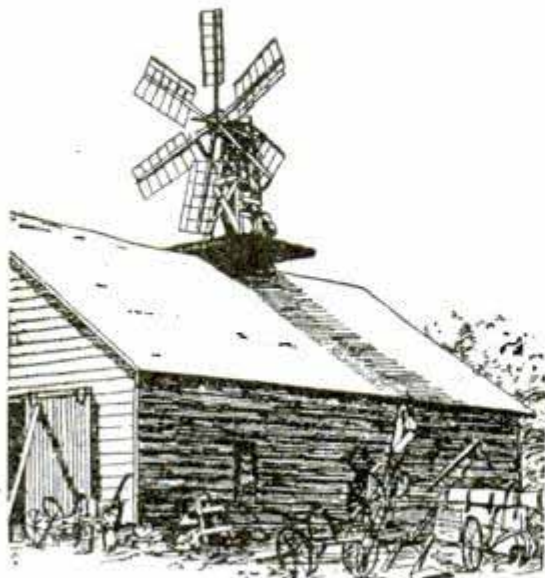
Fig. 12--Six-Fan Holland Mill
