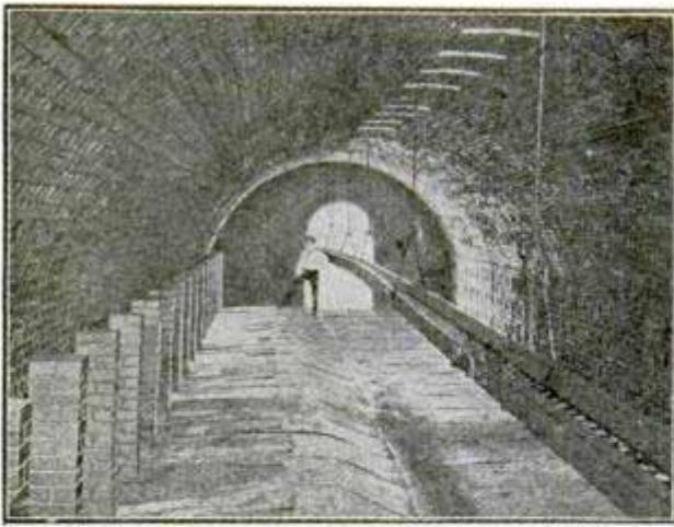
First Course Laid
