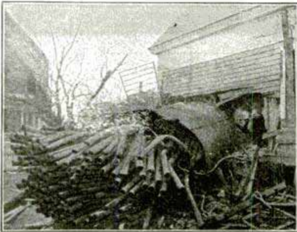
Brockton Lap-Joint Explosion--Boiler Was Hurled 215 Ft. and Moved House 16 In.
