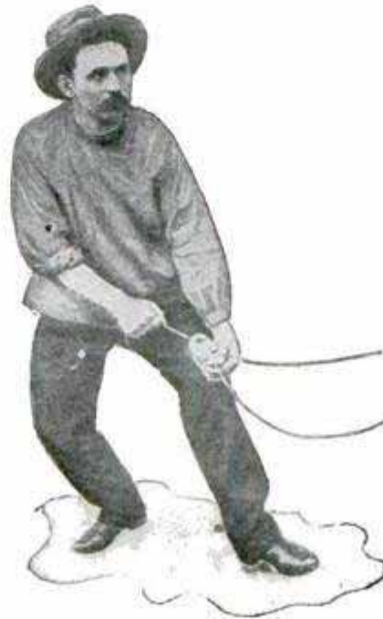
Setting Off the Blast
