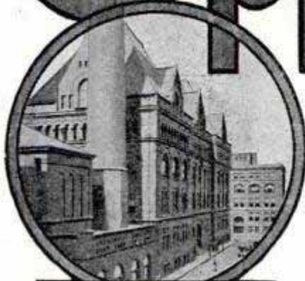
MAIN BUILDING ARMOUR INSTITUTE
