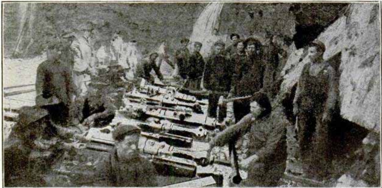
Battery of Air Drills Inside Cofferdam
