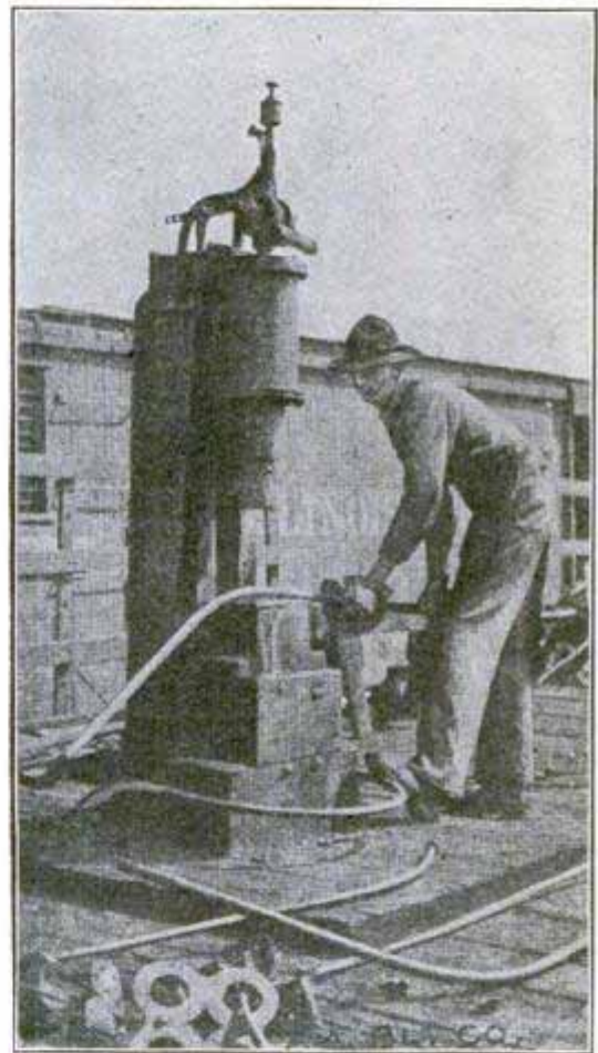
Air-Hammer for Straightening Scrap Iron.
