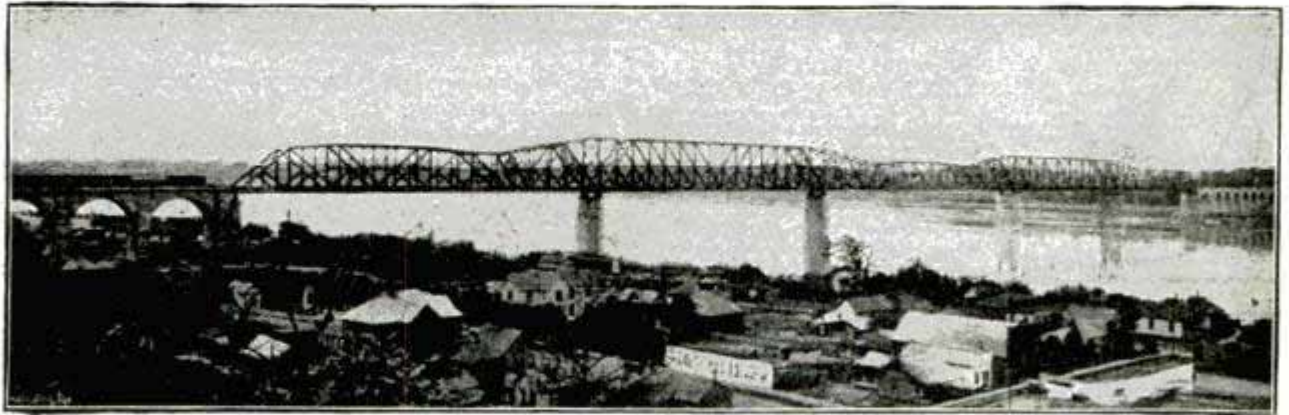
Thebes Bridge, 3,817 Feet Long--Ralph Majeska, Engineer.
