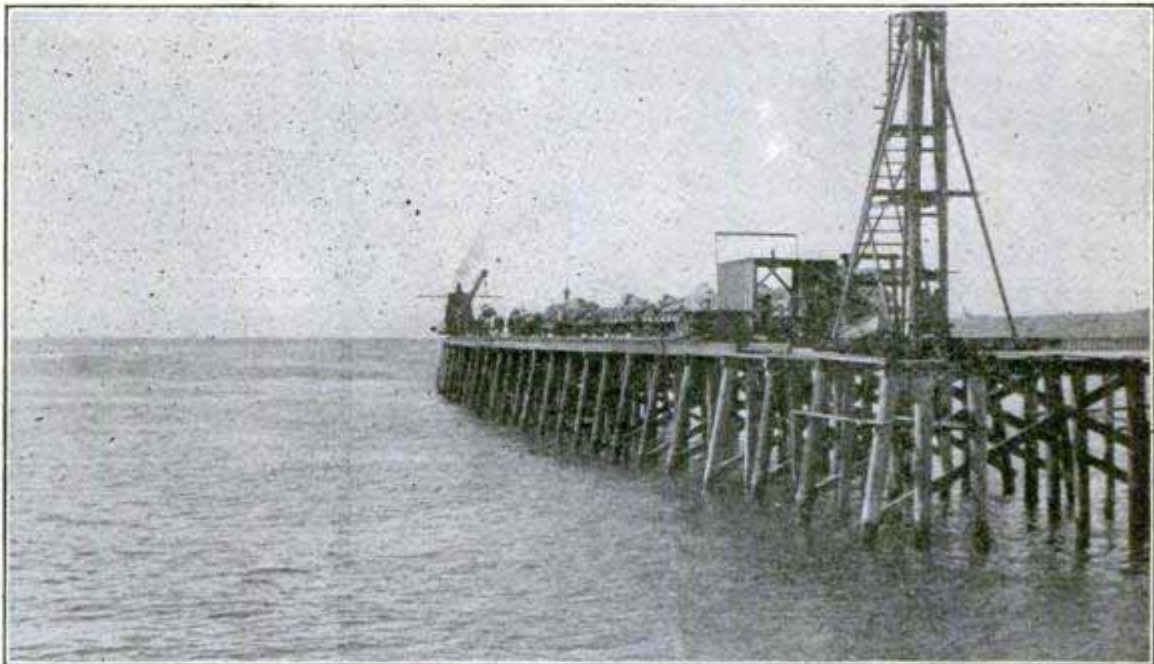
Building the Largest Breakwater in the World.
