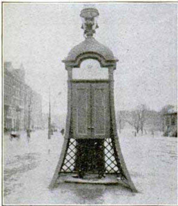
Telephone Pavilion Closed.
