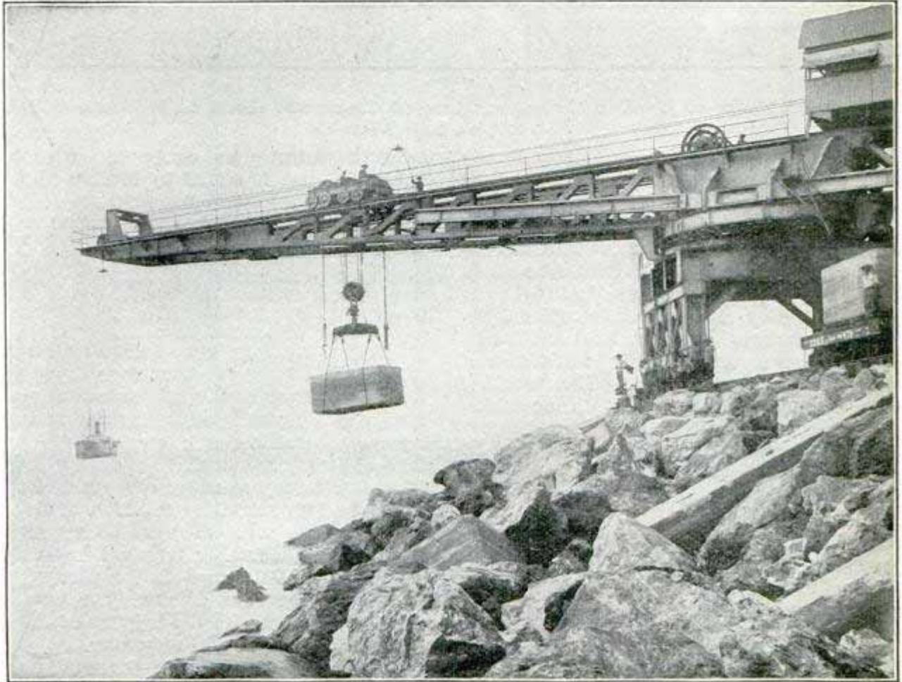
Immense Electric Crane Used in Building the Breakwater
