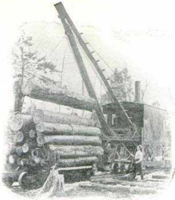
Log Held Steady While Loading by Tongs at Each End
