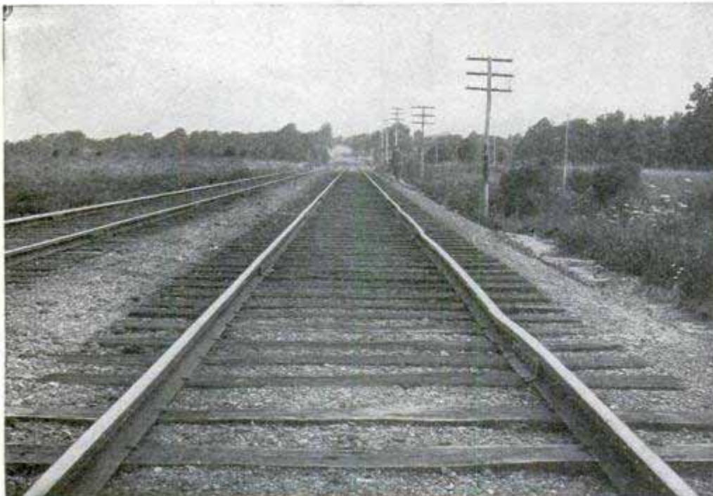
Rail Depression Caused by Imperfectly Balanced Locomotive
