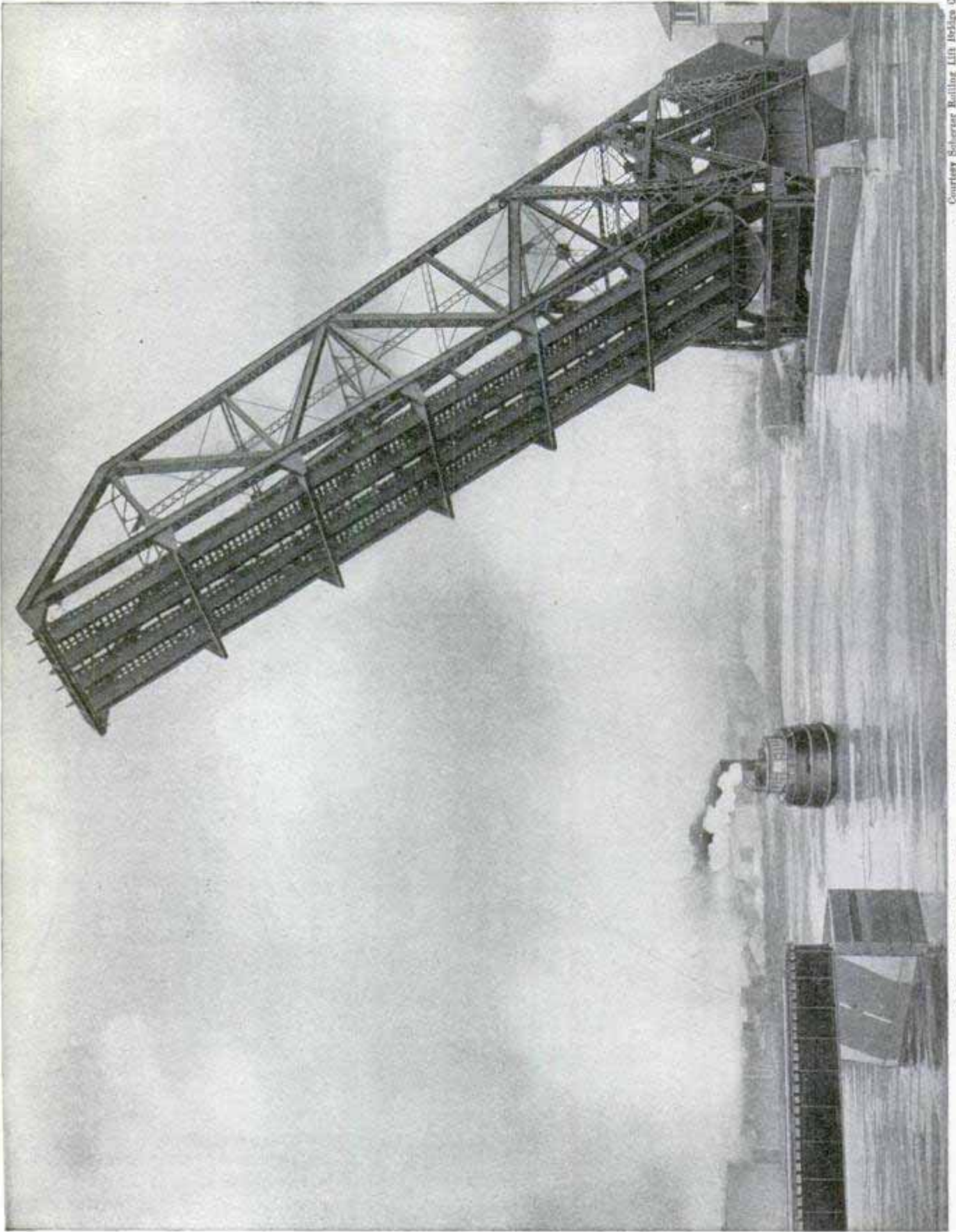
This Bridge Has a Single-Leaf Simple Truss Span 160 Feet Long
