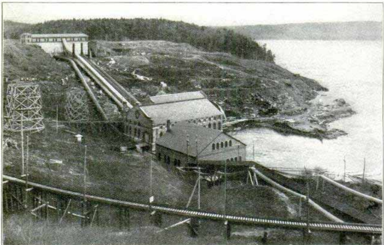
Head Race, 125 Feet Above the Power House
