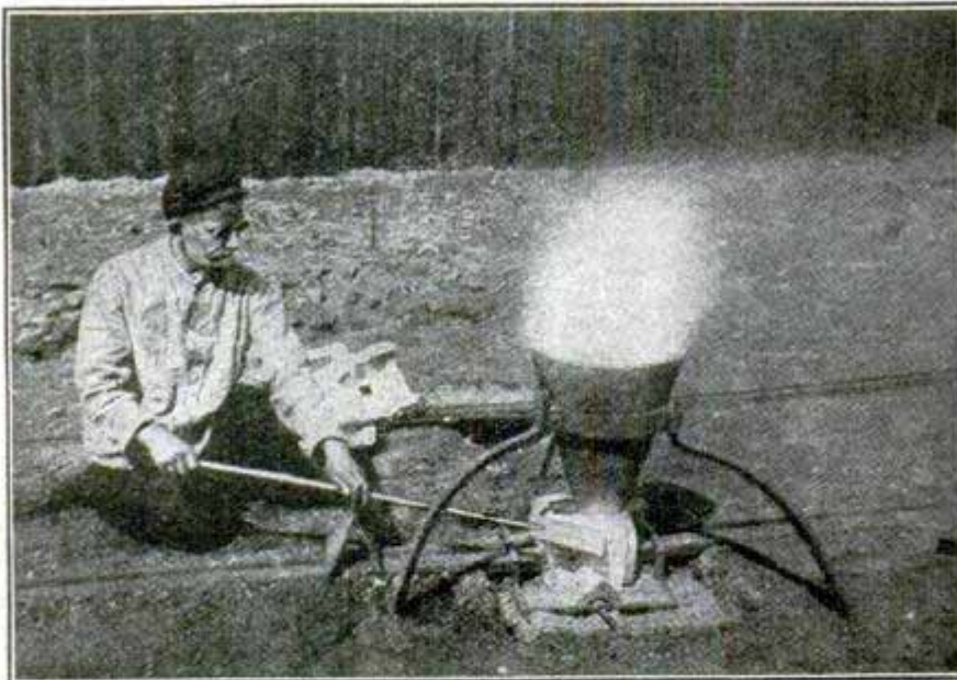
Fig. 4. Welding Without Clamps
